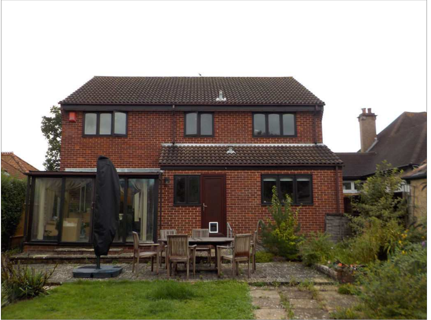
Rear of No. 25a Lovedean Lane
