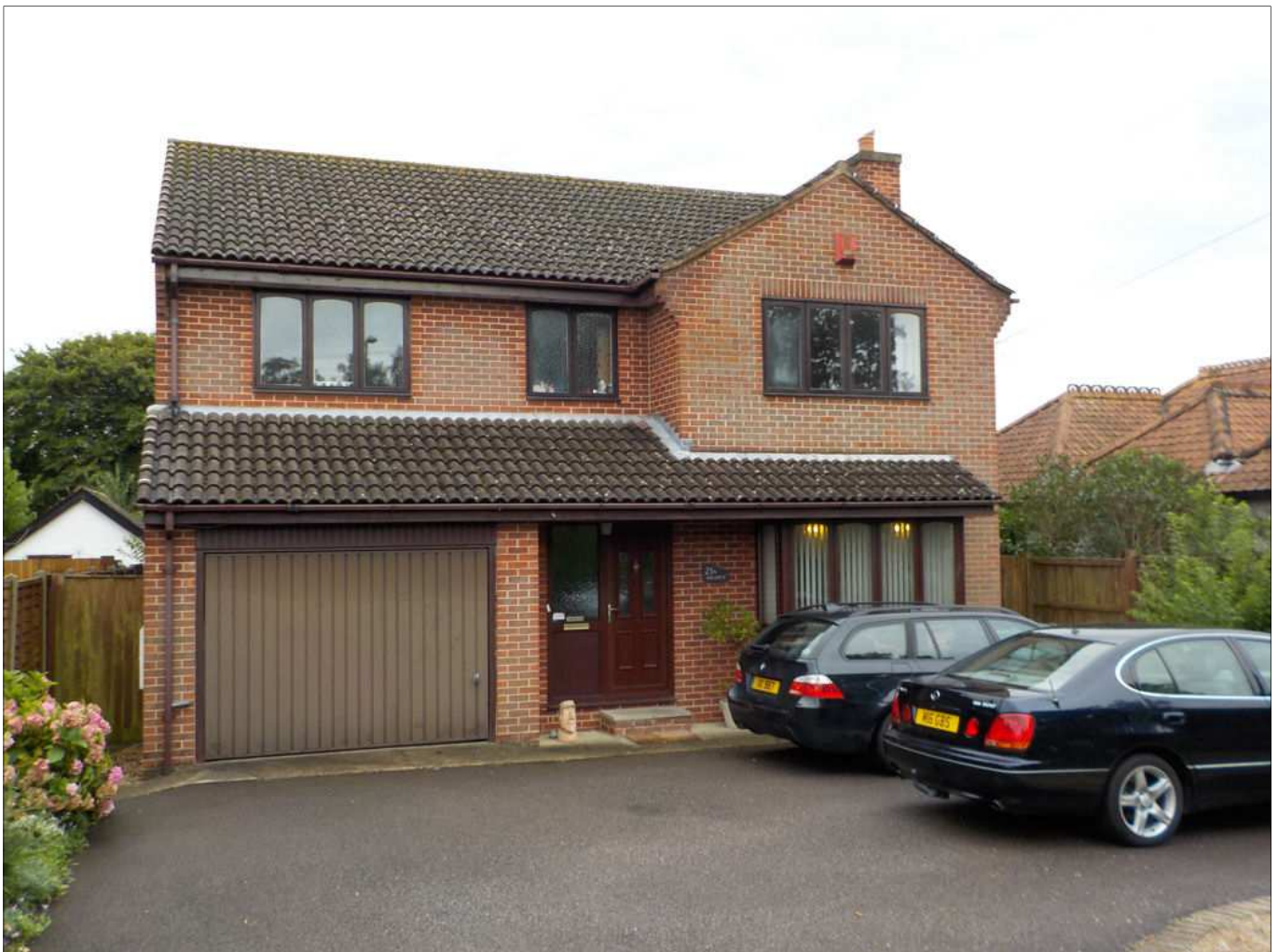
Front of No. 25a Lovedean Lane - no changes
