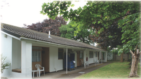
Typical examples of Accommodation Buildings
