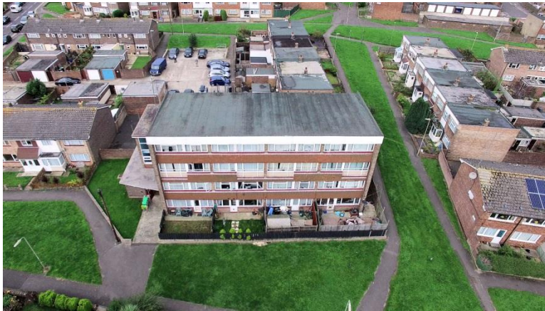
Photo 1 - Arial view of the block (Front Elevation)
