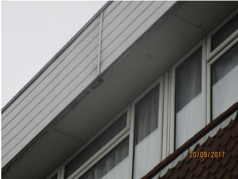
Photo 4 - Existing Facia Board and Soffit
