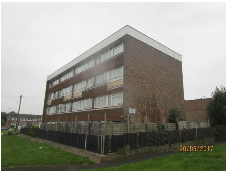
Photo 2 - Front Elevation showing boundary fencing
