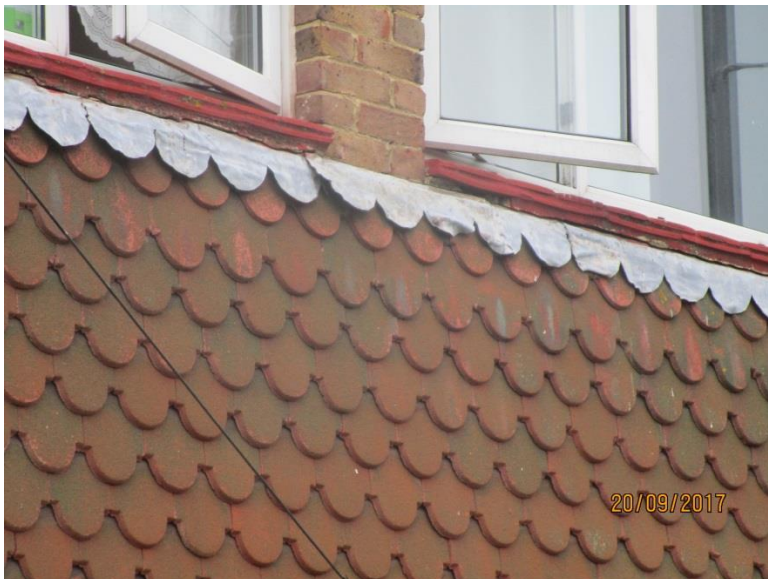
Photo 5 - Tile hanging to front elevation
