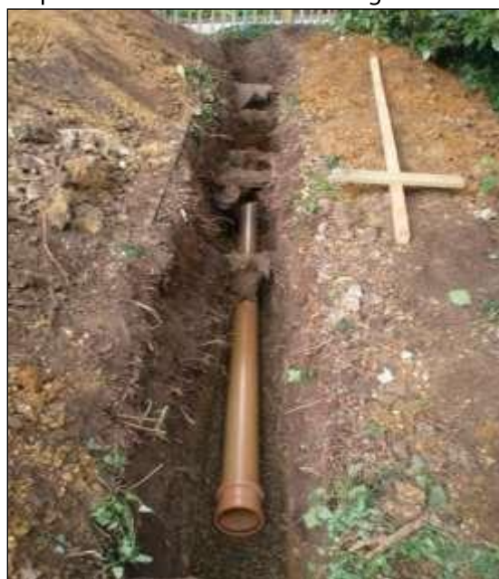
Services image 2: Continuous trenches dug by hand so that important roots can be retained (with the service ducting threaded beneath) is an effective means of minimising damage (note the ground protection boards with soil piled on top on the left).
