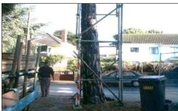
Fencing image 5: A scaffold-braced framework surrounding the trunk reduces the risk of accidental impact.
