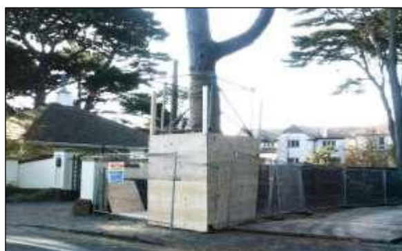
Fencing image 6: Board secured to scaffold framework adds another layer of protection for vulnerable trunks and branches
