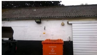
Plate 4.17: View of Building 13
