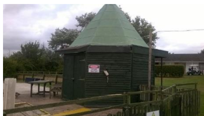
Plate 4.22: View of Building 1
