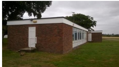
Plate 4.19: View of Building 42
