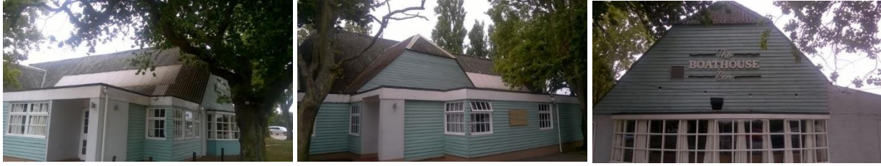
Plate 4.18: View of Building 11
