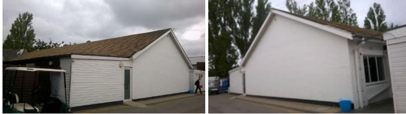
Plate 4.16: View of Building 12
