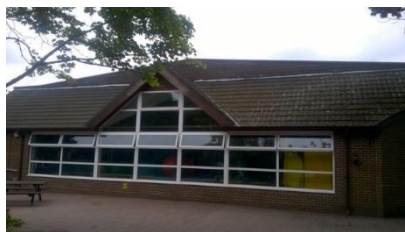
Plate 4.14: The western gable end of Building 10 with a large pitched roof with interlocking clay tiles and wooden cladding
