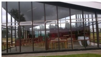
Plate 4.21: View of Building 49
