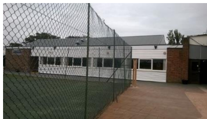
Plate 4.12: Southern extension of Building 9
