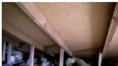
Plate 4.5: Boarding was present between the rafters and the roof tiles
