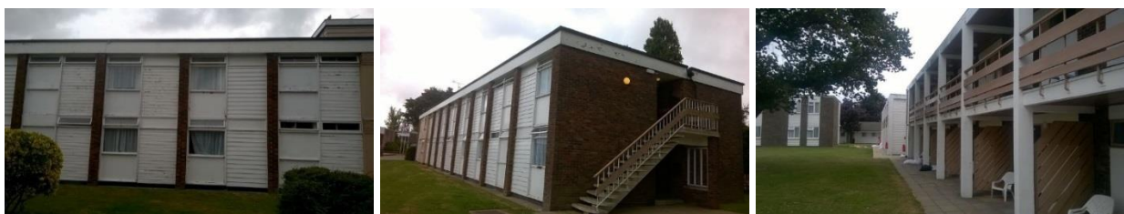
Plate 4.7: Example of the two storey accommodation units
