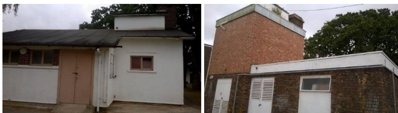
Plate 4.9: Example of the boiler houses
