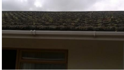
Plate 4.2: Roof tiles and walls in good condition
