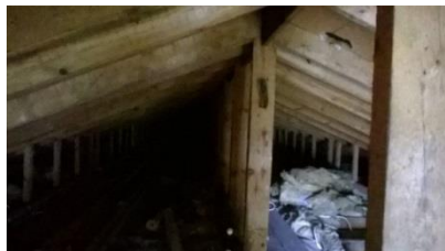
Plate 4.4: Internal view of the loft spaces
