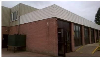
Plate 4.11: View of Building 9
