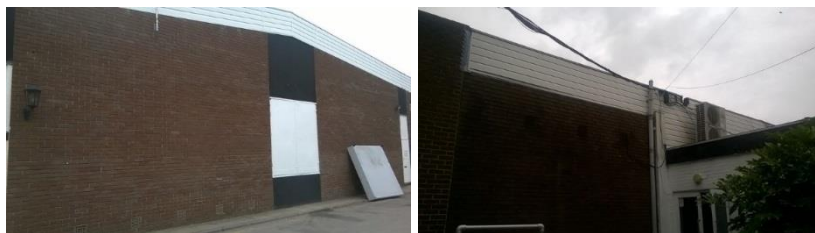
Plate 4.13: View of Building 10
