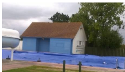
Plate 4.20: View of Building 48
