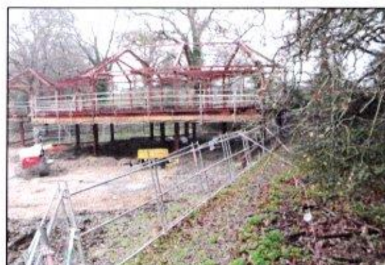
Photo 37: It is possible to support very large structures on piles within sensitive RPAs without any significant adverse impact on tree roots.
