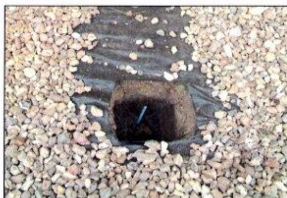
Photo 39: Ground protection must be used to spread the load of the piling rig once excavation has confirmed that no substantial roots are in the preferred pile location.
