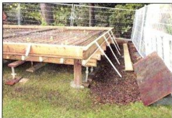
Photo 36: Small diameter piles (less than 150mm) are an effective means of supporting structures in RPAs with minimal disturbance.
