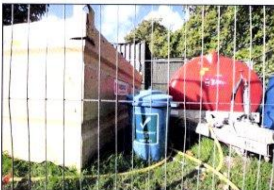
Photo 46: Where fuel or other chemical are stored on site, it is now standard practice to have emergency spillage kits available to restrict the environmental impact of accidents.
