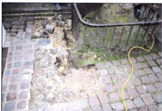
Photo 21: Careful lifting of cemented-in sets round this tree allowed them to be re-laid on a permeable sand base, improving the water input into the soil around the trunk.
