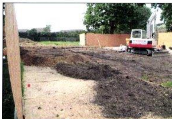
Photo 8: Spreading soil excavated from footings is an effective way of buffering the plywood surface from the wear of light vehicles.
