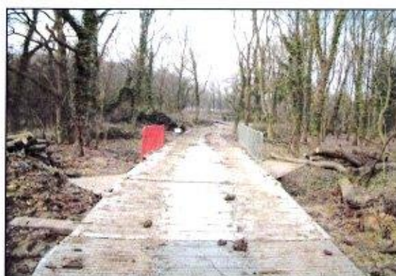
Photo 12: Custom designed sectional tracks can be joined to support very heavy traffic use through sensitive areas.
