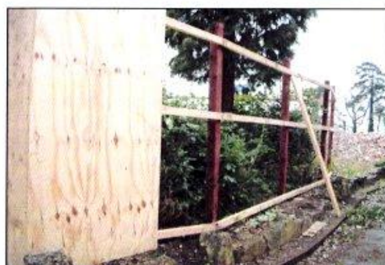
Photo 4: Board specification on secure wooden posts is a suitable alternative to the standard braced scaffold design.
