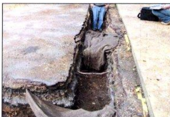
Photo 18: Exposed roots must be protected from light, drying out and extremes of temperature by covering with hessian sacking and boards until they can be covered back with soil.
