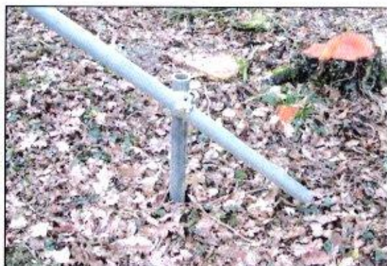
Photo 3: Close up of bracing detail, essential for increasing the stability of the vertical framework.
