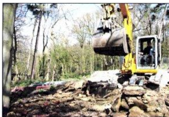
Photo 20: Machines with a long reach can be used to lift out heavy surfacing and structures as long as the machine sits outside the RPA and the exposed surface is protected before there is any further access.
