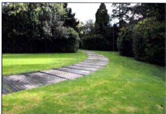
Photo 19: Ground protection must be used where repeated foot or vehicle traffic could cause compaction in sensitive RPAs. It can be as simple as plywood for pedestrians, but must be more robust for vehicles.
