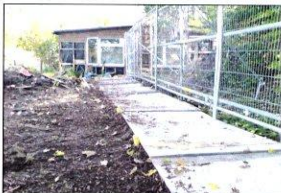
Photo 7: Heavy-duty plywood set onto a compressible woodchip layer and pinned into position is suitable to spread the loading from pedestrian access.
