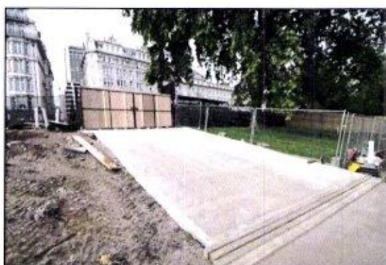
Photo 30: This temporary access for heavy construction traffic on the outer edge of a RPA is a concrete slab cast above ground level and will be removed when the project is completed.
