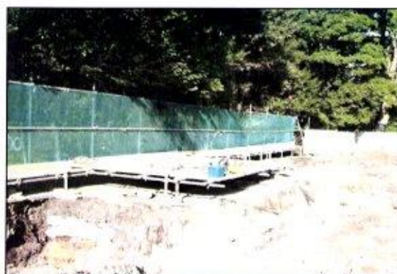
Photo 10: A scaffold framework attached to the main scaffold fencing can be used to support either scaffold planks or plywood to create an elevated platform with a gap beneath.
