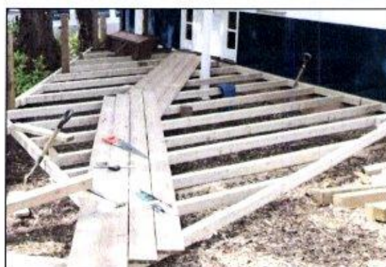
Photo 35: This deck supported above the ground on small posts provides a low-impact alternative to conventional stone patio surfacing in RPAs.
