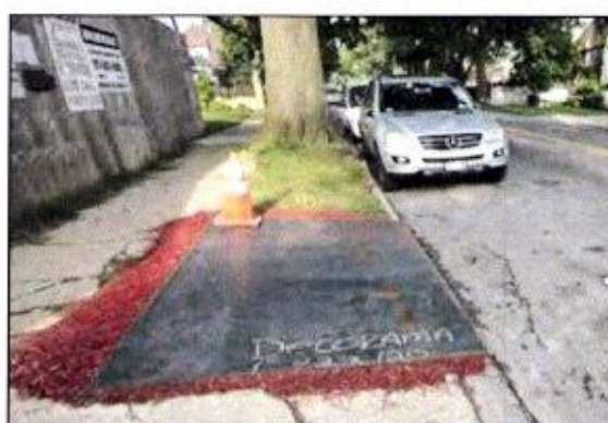
Photo 14: Steel plates can be an effective way of temporarily reinforcing weak surfacing over a construction access during the development activity.
