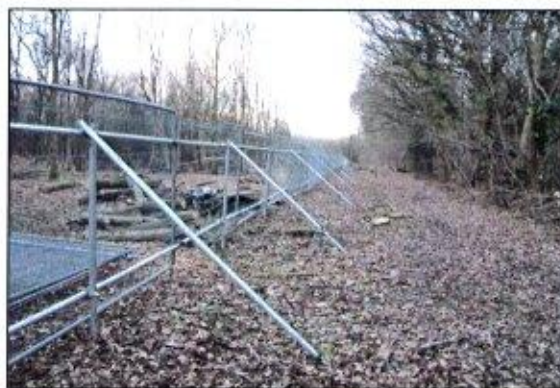
Photo 2: Heras fencing wired to scaffold braced posts is a robust and effective interpretation of the BS specification.
