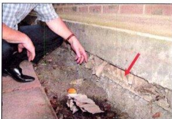
Photo 42: Where a slab is cast on site, a biodegradable void-former (red arrow) temporarily supports the weight of the liquid concrete until it sets. The void-former can then be wetted and washed away to leave a void or left to degrade naturally, both of which allow movement of air beneath the slab.
