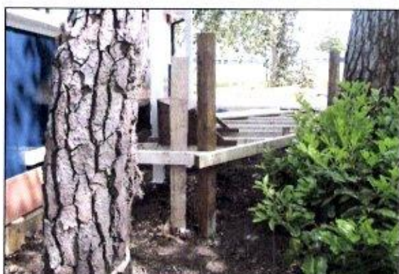
Photo 32: New surfacing can be supported above the ground on posts leaving the soil surface beneath undisturbed.
