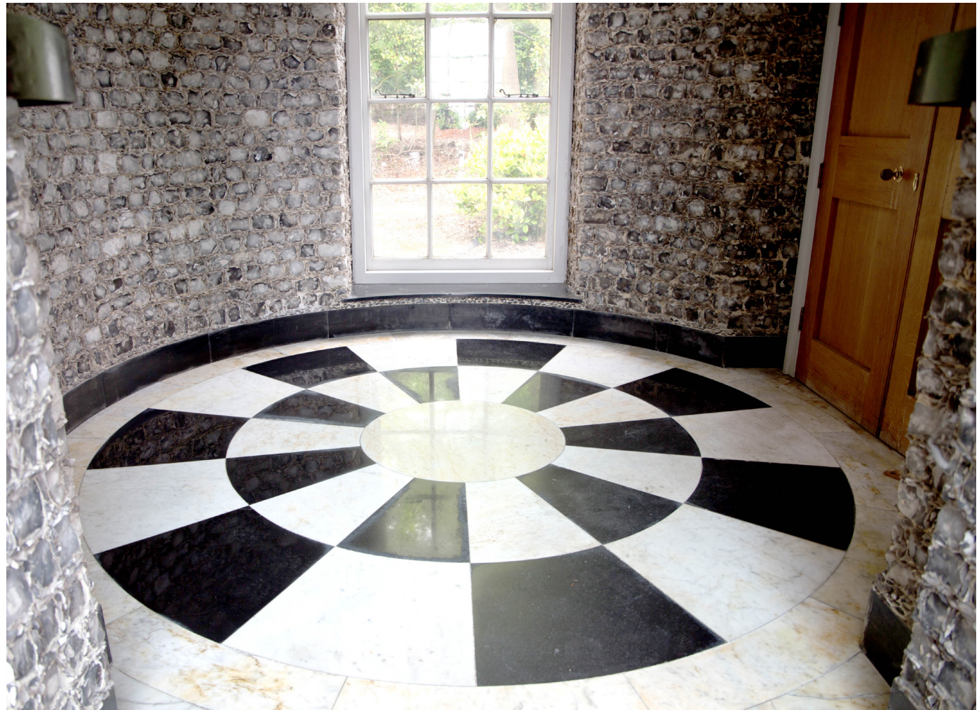
Decorative marble floor to entrance lobby
