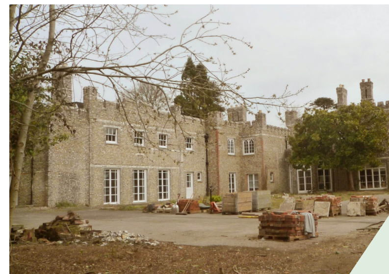
Main house during renovation
