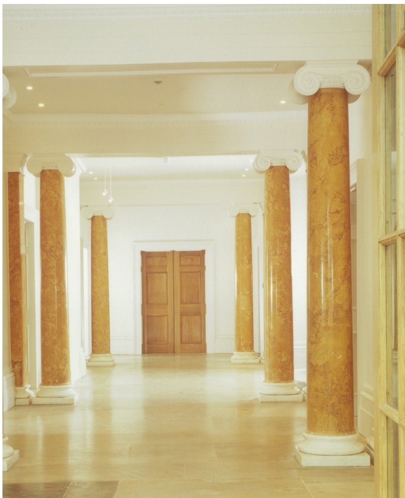
Scagliola columns to main corridor
