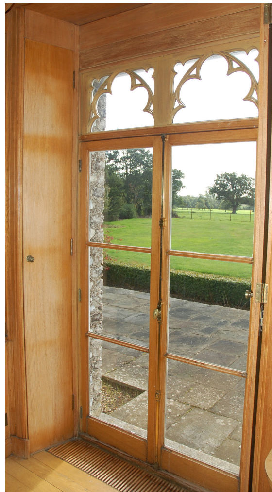
French windows to library with shutters to reveals
