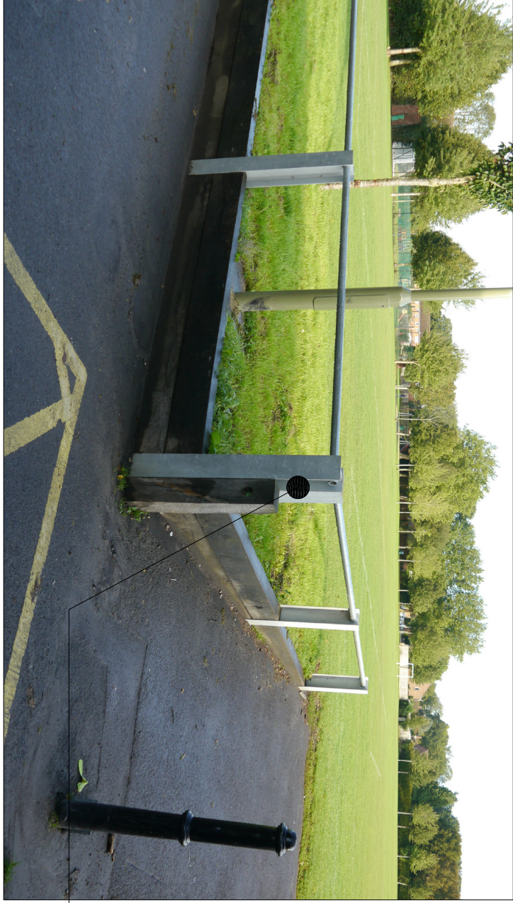
Existing Steel posts and sleepers to be carefully removed and reused as retaining wall for additional parking area
