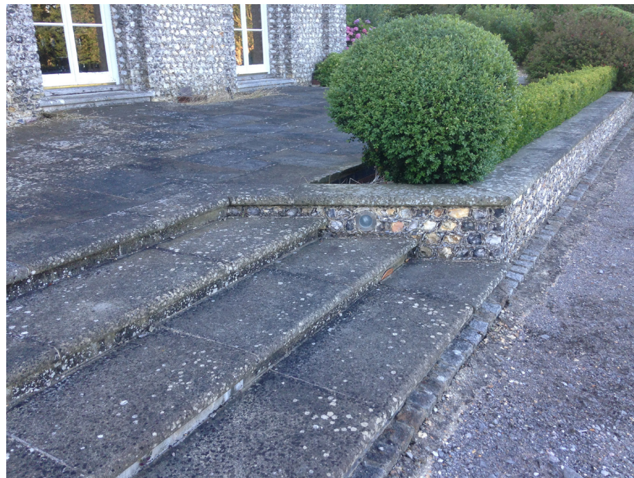
Photograph S4. From south terrace of Southleigh Park House
