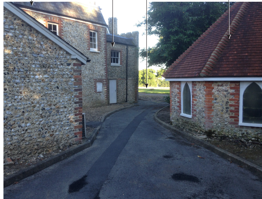
Photograph S5. From site road on east side of house
