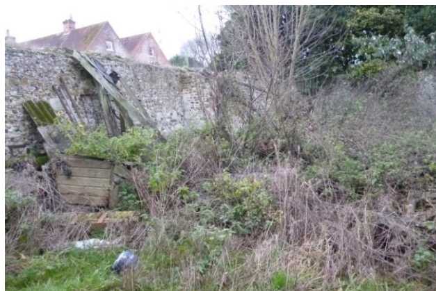
Figure 9 – Existing east gable wall permitting access for wildlife.
