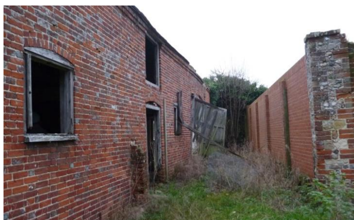
Figure 3—South elevation of stables facing west (entrance to site)
