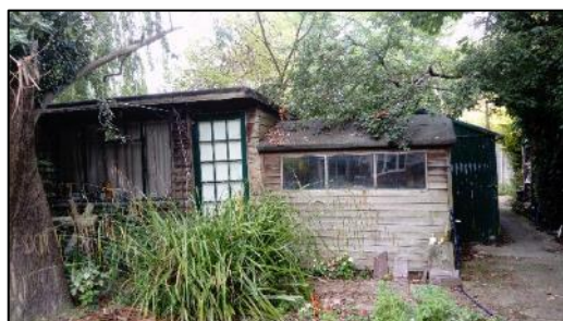
Figure 1: South-eastern elevation of studio accommodation (left) and adjoining shed (right)
