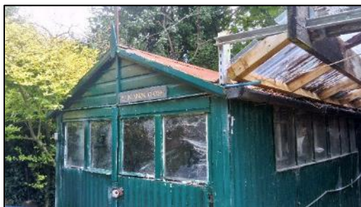
Figure 3: Eastern elevation of tin garage
