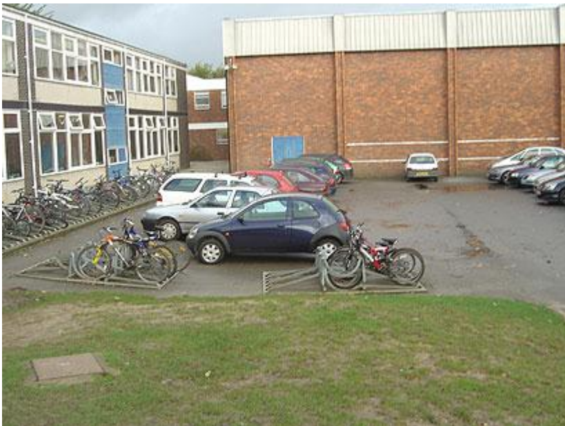
Cycle storage area, at the rear of school
