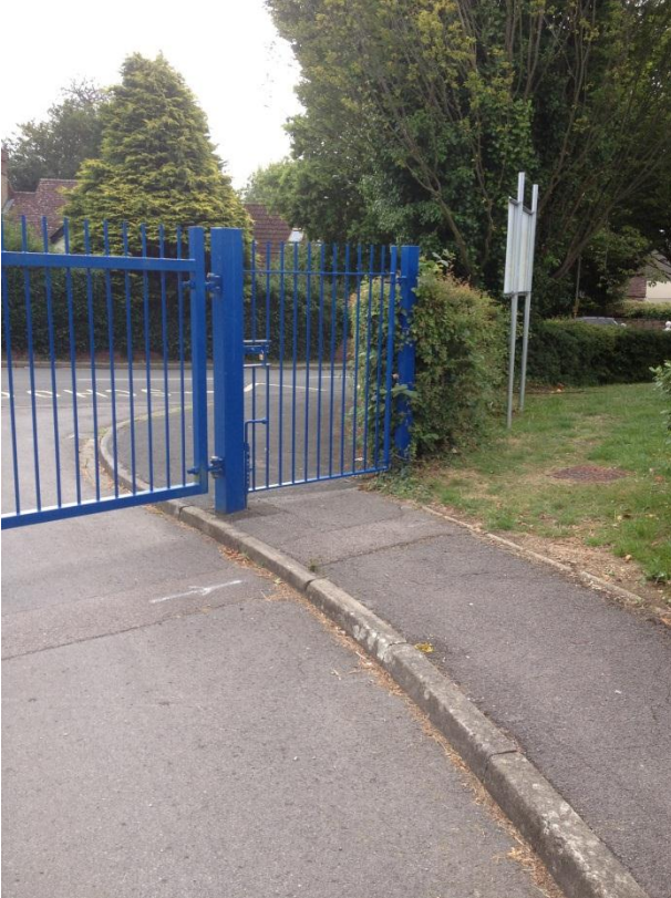
New vehicular and pedestrian gate at the rear access to school
