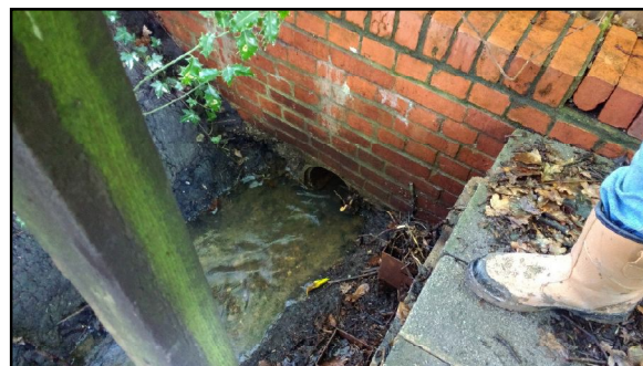
Figure 2.3. Church Road Stream Headwall
