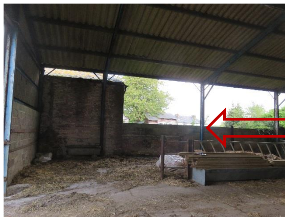
Interior of Barn (1 st Two Bays Removed)
