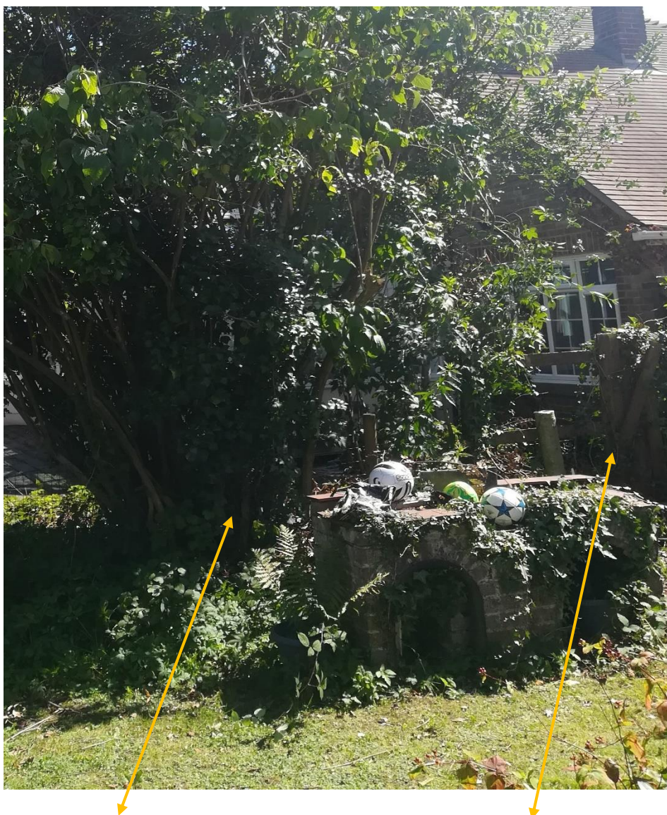
Lilac encroaching into neighbouring land.
