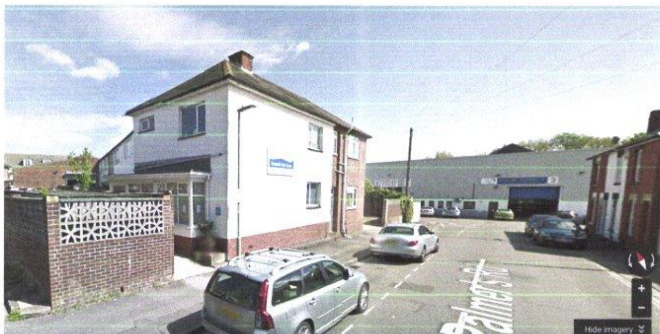
Image 6: Existing signage on south facing aspect of building.
