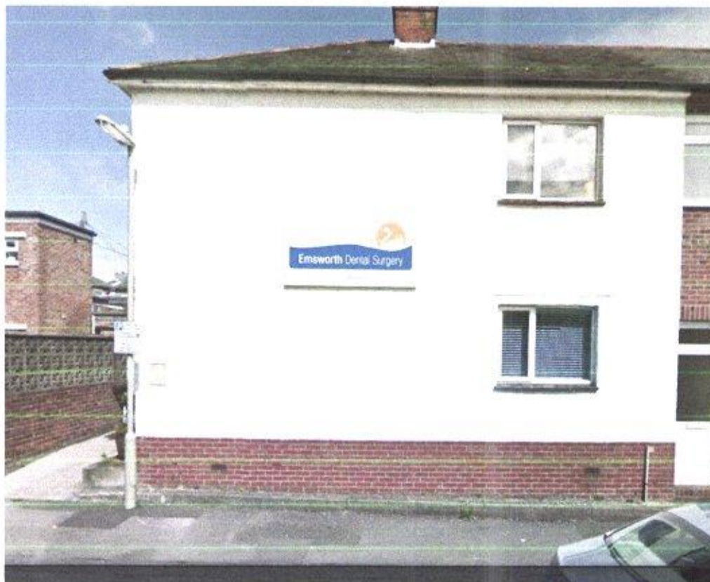
Image 5: Existing signage on south facing aspect of building.
