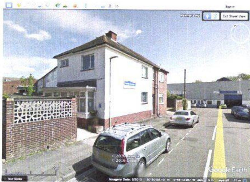
Image 1- Existing signage on south east aspect of building to be replaced by proposed new signage.
