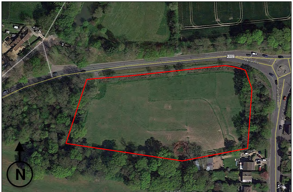
Figure 2.1. Aerial view of the plot
