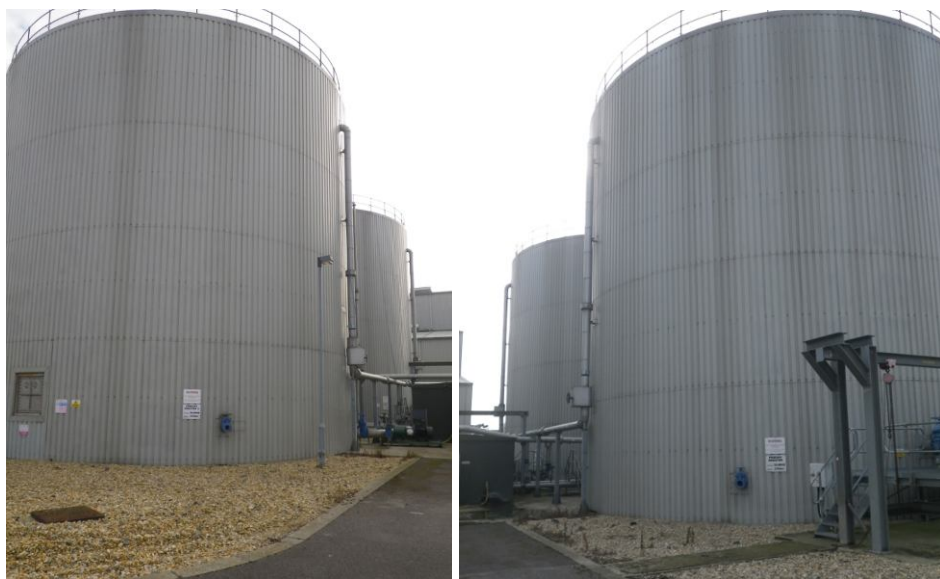
Figure 2: Existing Digester finish to be replicated.
