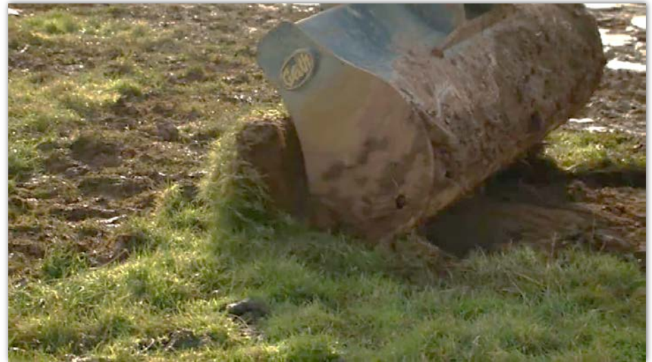
Figure 12. Top Soil Stripping
