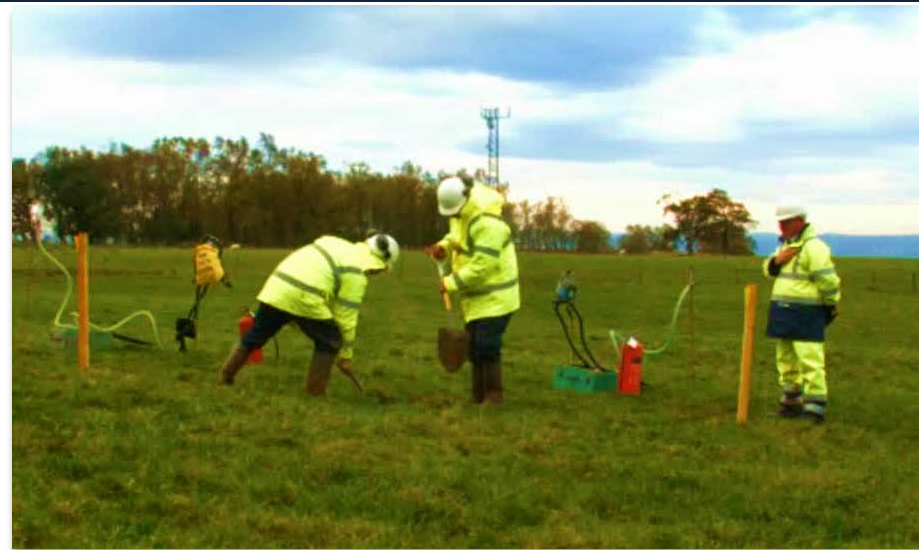
Figure 4. Hand Excavated Trial Hole
