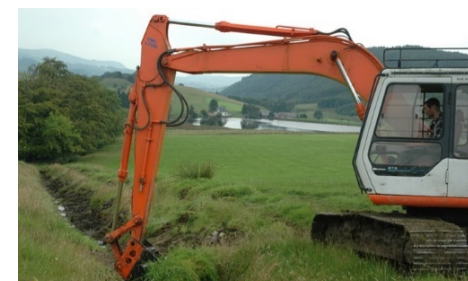
Figure 2. Ditch Maintenance
