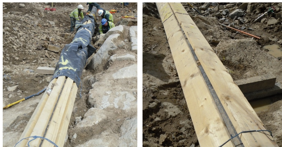
Figure 14. Protective cladding applied to pipeline
