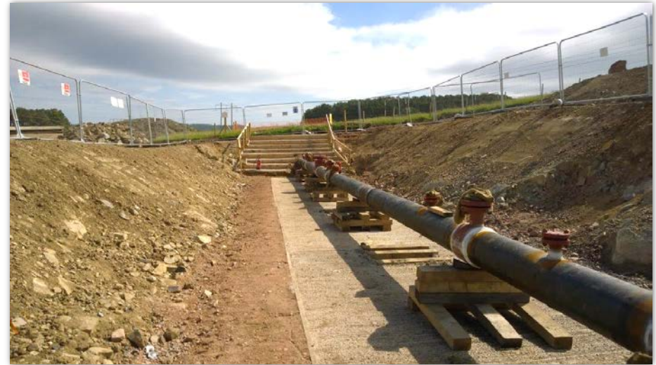
Figure 20. Pipeline Supports
