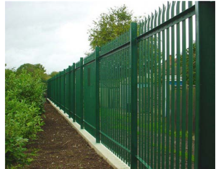
Typical 2.4m high palisade fencing in Green RAL 6005
