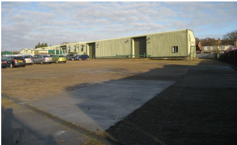
Unit 2 and Forecourt
