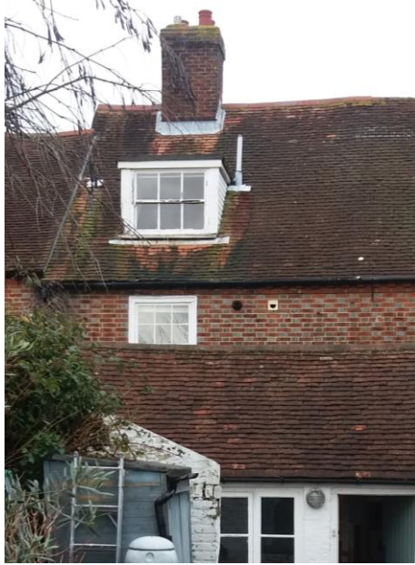
View existing dormer window from the rear garden
