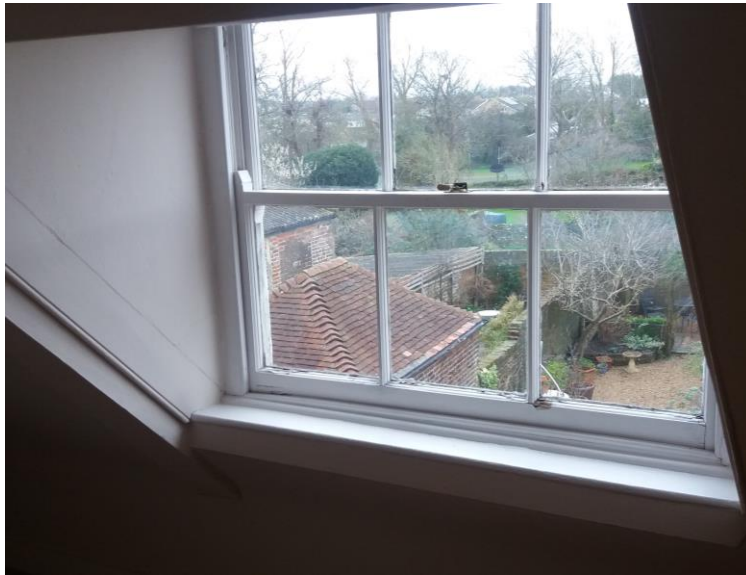
Internal view of existing windows
