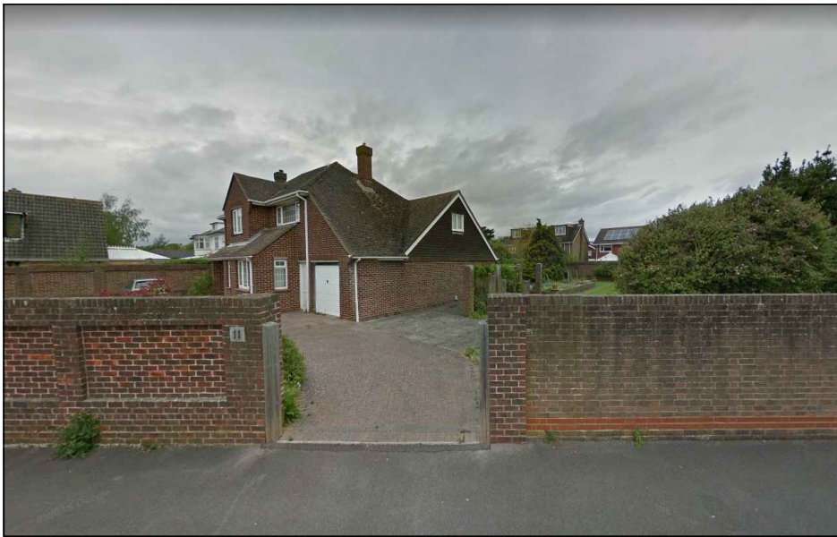
VIEW OF EXISTING VEHICLE ENTRANCE
