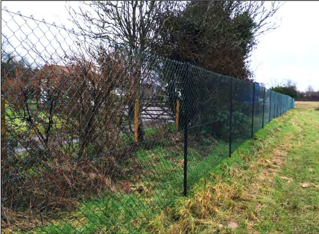
Chain-link on angle-iron uprights
