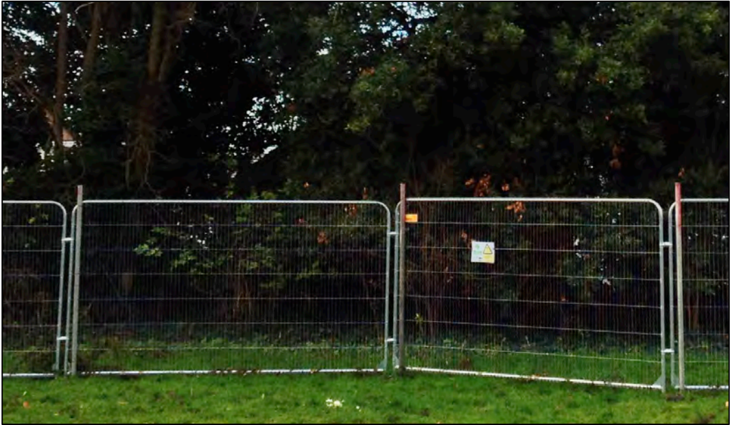
Weld-mesh panels on scaffold uprights
