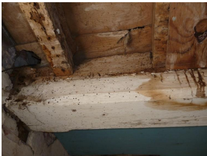
Figure 28 – Woodworm infected beam to be treated
