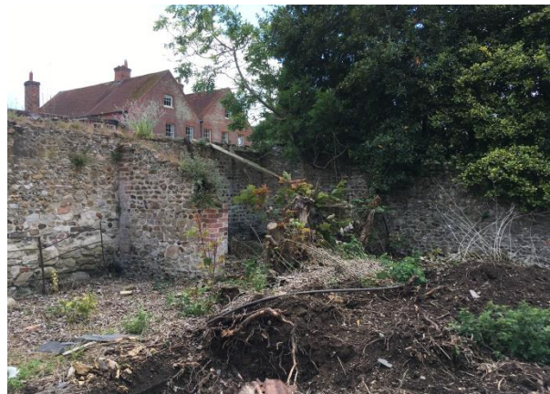
Figure 36 – Original remains of structure south of the garden to be retained
