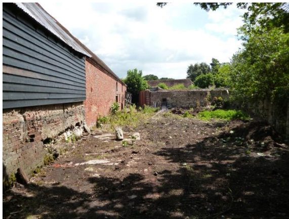
Figure 35 – Entrance to site with paving running the length of the barn to be relayed for level patio.
