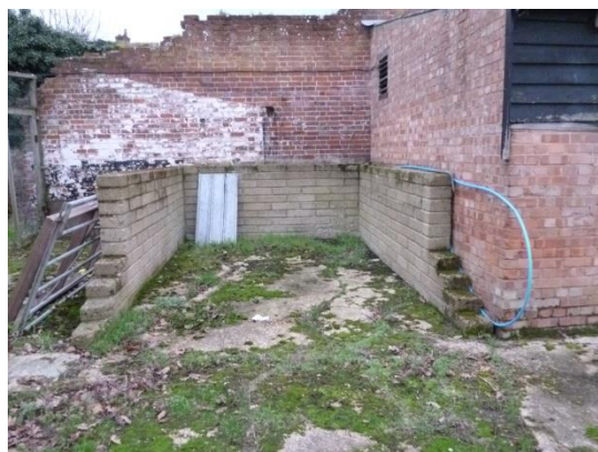
Figure 13 – Blockwork to be removed
