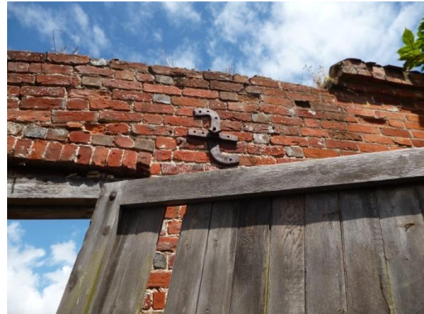
Figure 4 – redundant reinforcing S shaped tie rods to be stored and re-used
