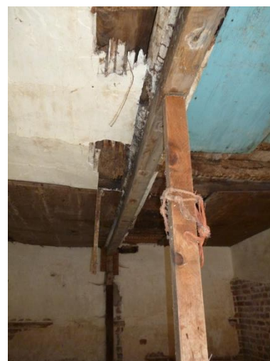
Figure 29 – Reinforcing wooden posts to be removed
