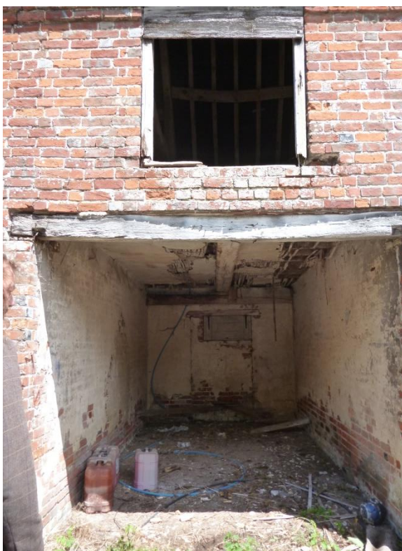
Figure 21 – Wide opening and hayloft opening above.
