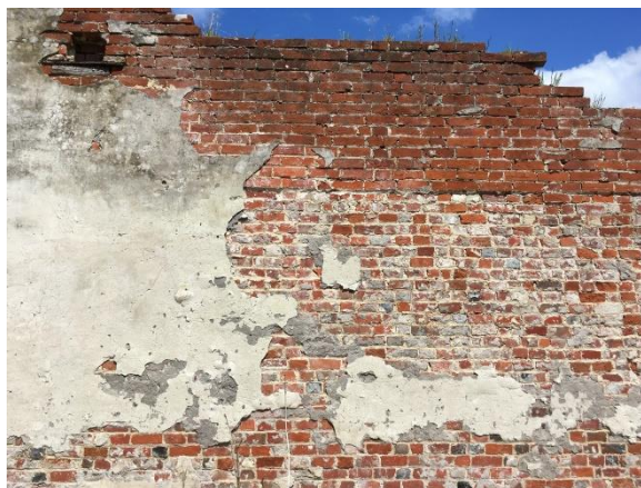
Figure 2 – Roofless wall to be retained on North elevation.
