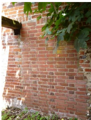
Figure 33 – Remove brick work to re-introduce opening.
