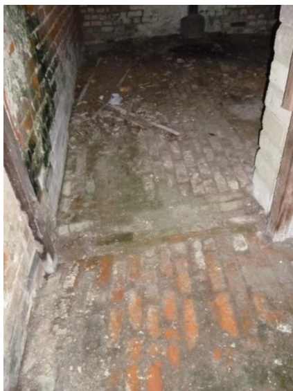
Figure 22 – Internal original brick paving
