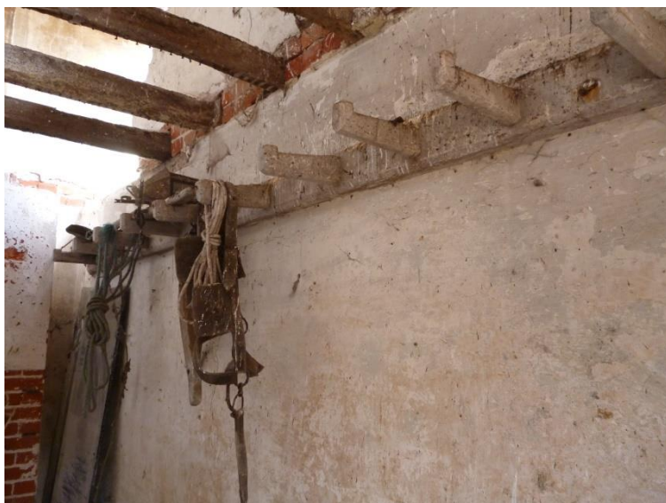
Figure 39 – Hanger to be salvaged and re-used
