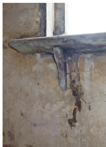
Figure 16 – window boards for re-use
