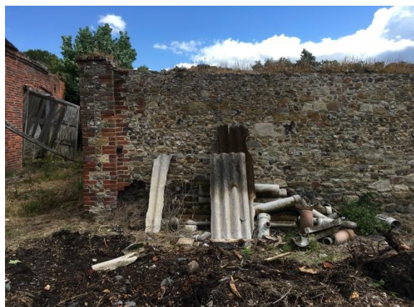
Figure 31 - Debris to be removed.
