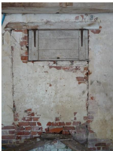
Figure 15 – Doorway to be re-opened
