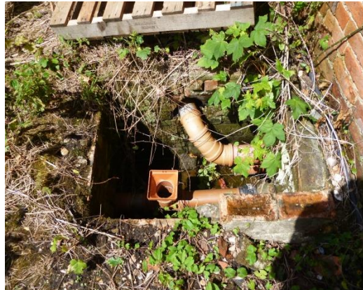
Figure 34 – Drainage hole to be covered
