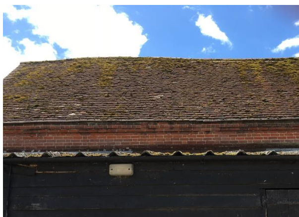
Figure 10 – Existing roof covering to be retained in part.
