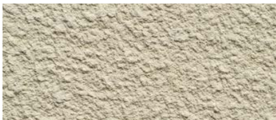
Monocouche off-white colour roughcast finish
