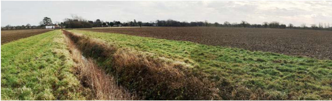
1. View of site looking east along culvert towards Hordean Road
