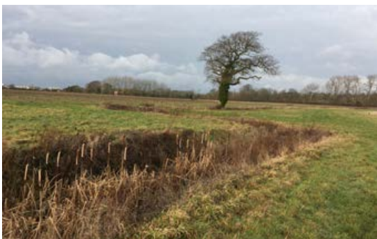
7. View looking north along culvert towards significant tree
