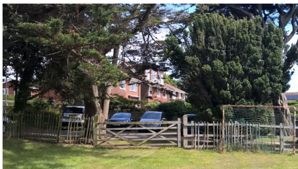
Residential properties east of site
