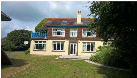
Existing building on site
