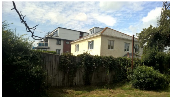
No.384 and Channel House west of site
