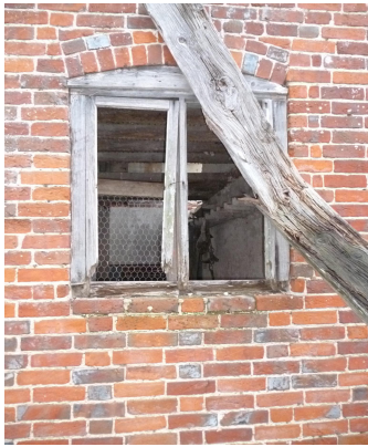
Fig. 5 - cambered openings
