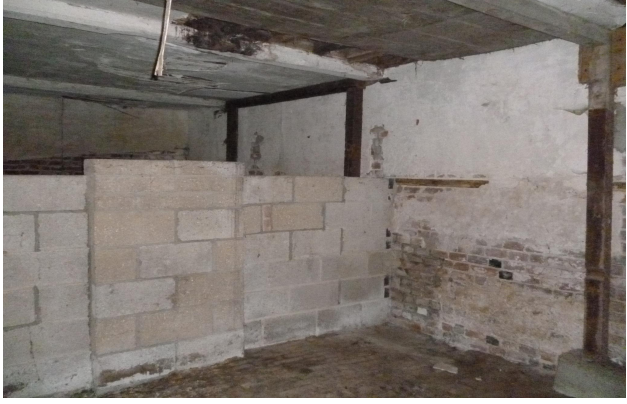
Fig. 4 - sub dividing concrete blockwork. Supporting steel posts
