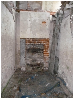
Fig. 6 - original brick chimney
