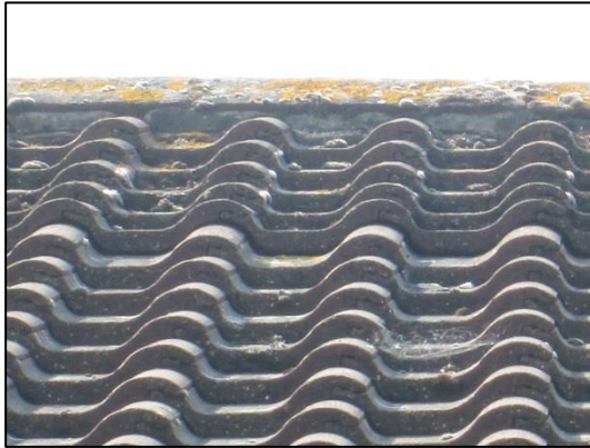
Figure 7 (left): Raised tiles found throughout building on pitched roof
