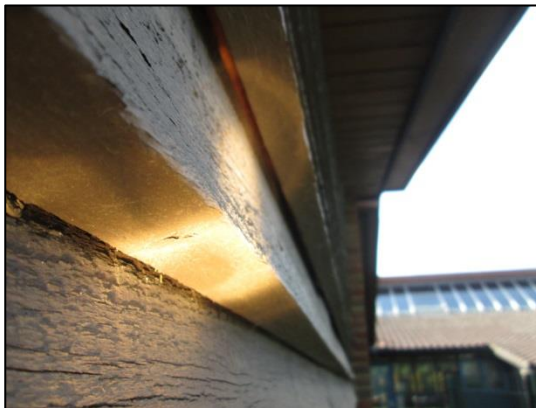
Figure 9 (left): Loose wood cladding on western elevation
