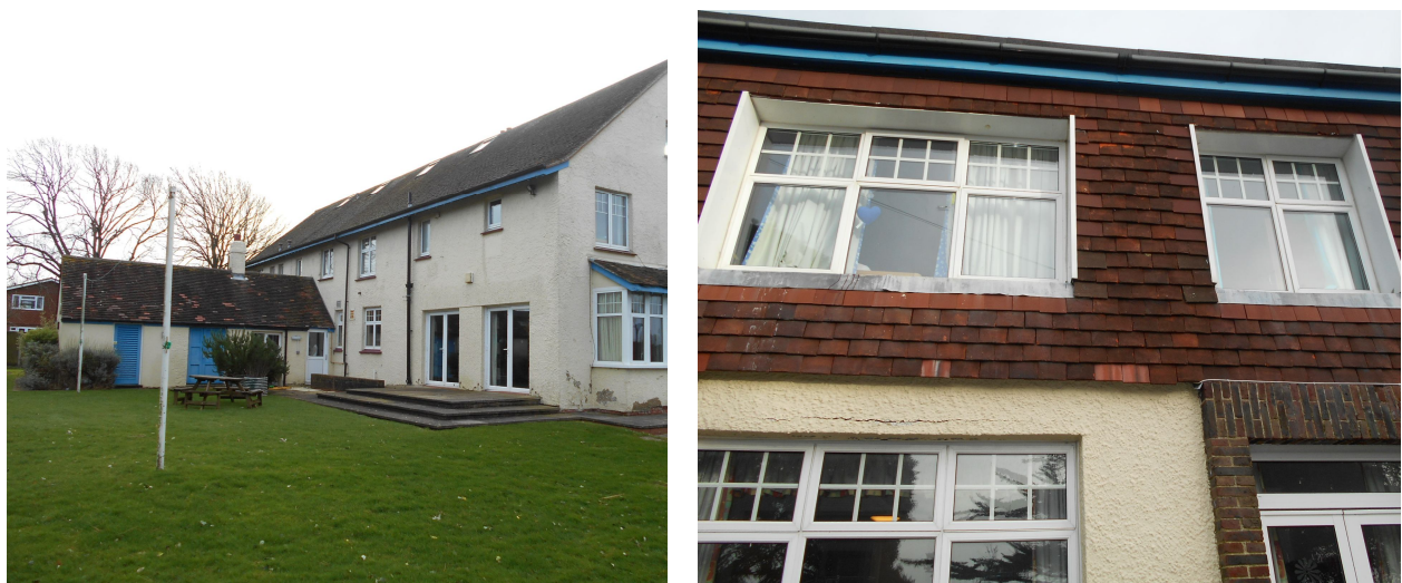
Figure 1: (left) Showing the northern elevation of the building and (right) showing the extension to the south of the building. No evidence of roosting bats was identified in the roof voids, but
