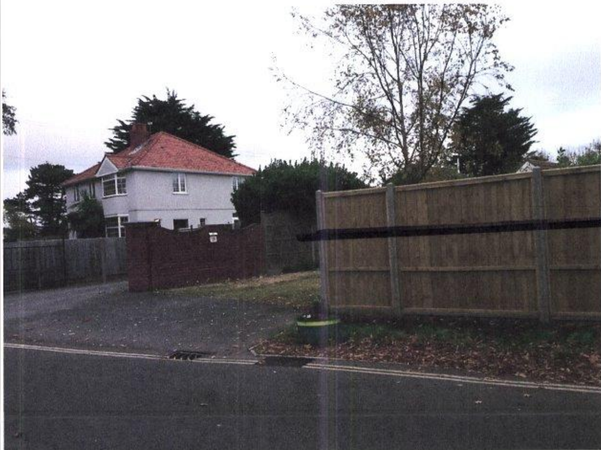
(1) Drive entrance and first 2 panels
