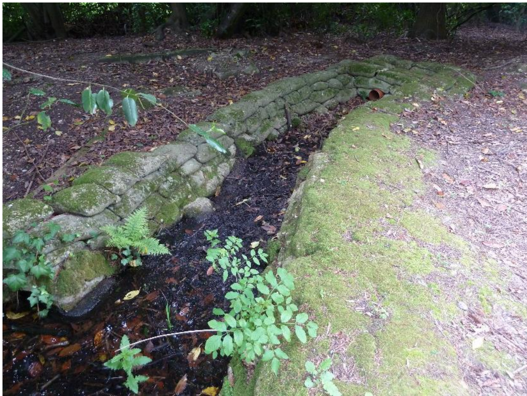
PHOTOGRAPH J: The Pond Outfall, looking south-west
