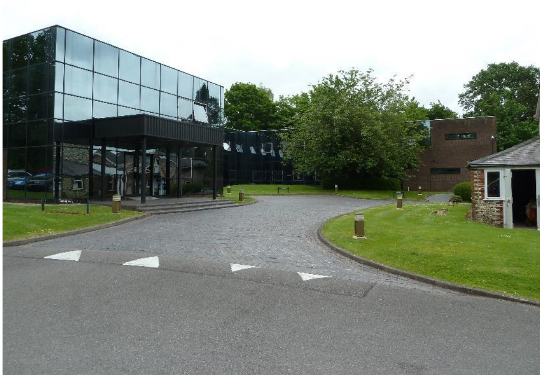
PHOTOGRAPH A: Main Office Building Entrance, looking northeast from the Eastleigh Road vehicle access
