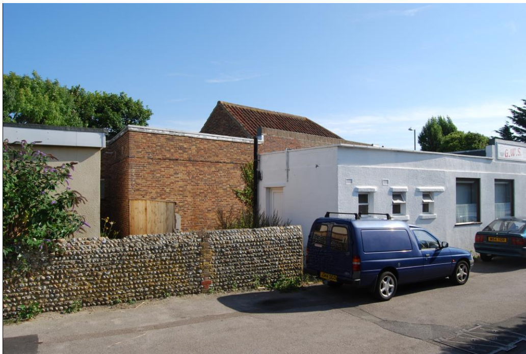
View of the existing South Elevation from the 65 Manor Road adjacent building.
