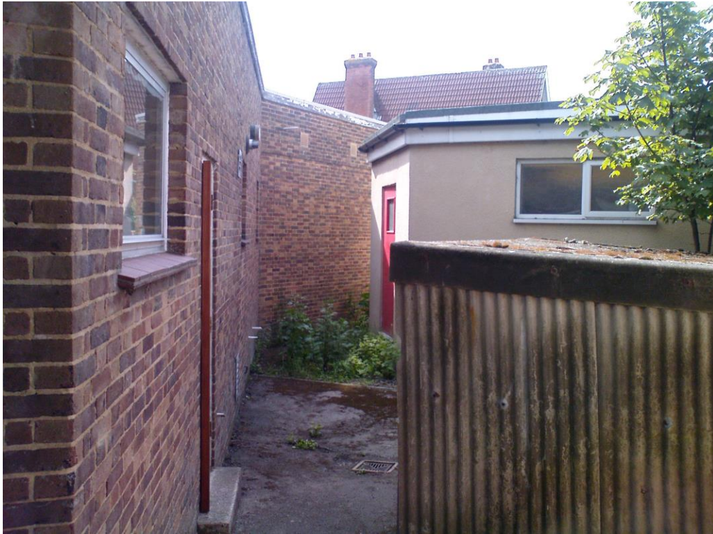
Existing West Elevation from the backyard.
