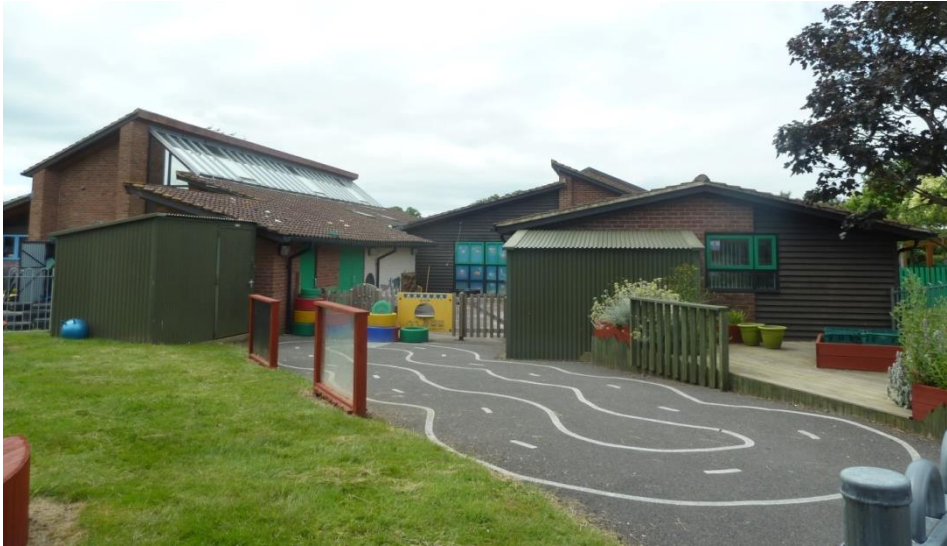
Trosnacc Children's Centre entrance and Trosnant Infant School
