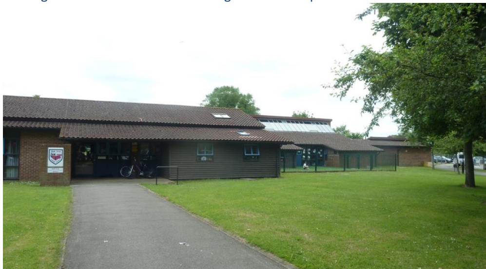
Former Junior school entrance (currently staff entrance)
