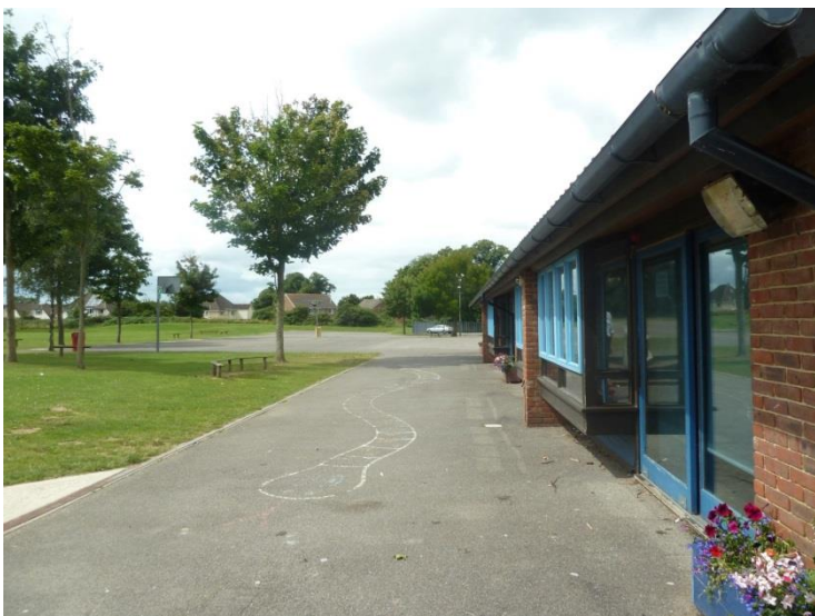
View from junior classrooms towards play court
