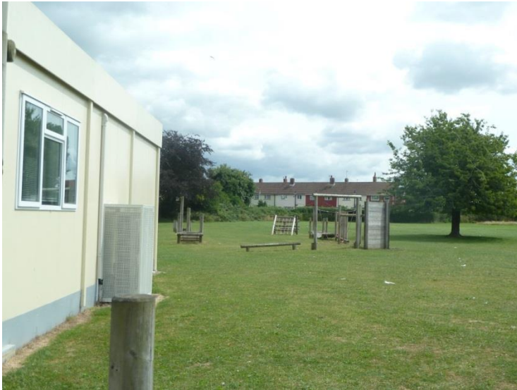
View of the temporary classroom towards the playground
