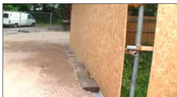
New surfacing image 5: Although this is only a temporary surface, railway sleepers pinned into the ground can be used to retain the edges of new surfacing.
