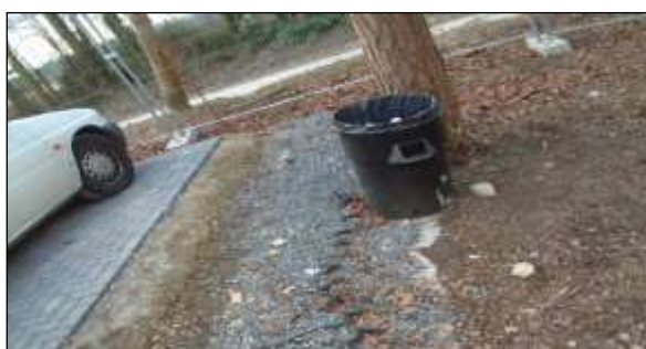
New surfacing image 4: A conventional concrete haunching can be used to retain new surfacing as long as it is not dug into a trench - here it is placed on top of the CellWeb layer.
