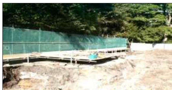
Ground protection image 4: A scaffold framework attached to the main scaffold fencing can be used to support either scaffold planks or plywood to create an elevated platform with a gap.
