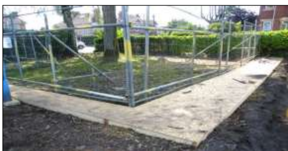
Ground protection image 3: Plywood fixed to a wood frame is another effective method of protecting soil from pedestrian compaction.
