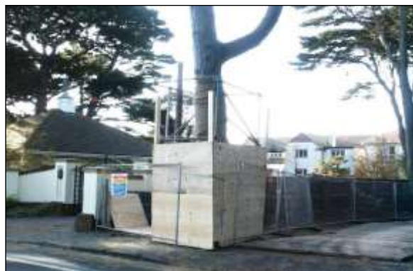
Fencing image 5: Board secured to scaffold framework adds another layer of protection for vulnerable trunks and branches
