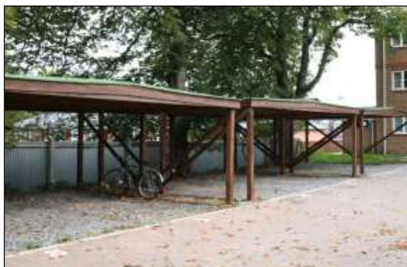
New structure image 1: These carports are formed by wooden posts above a three dimensional cellular no-dig and load-spreading surface of permeable crushed stone.
