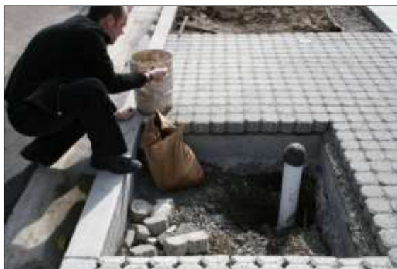
Soil cell image 3: The finished surfacing is profiled to leave the tree pit open, ready to be filled with good quality topsoil and the new tree.
