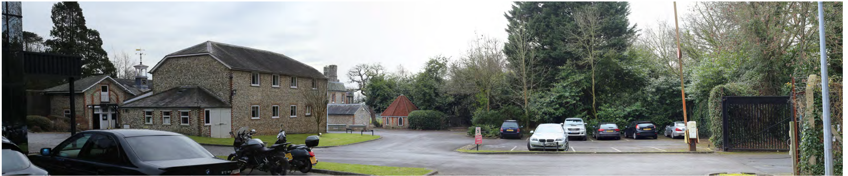
The former service courtyard showing the coachhouse, stable block with clock, and dairy with the offices and car parks
