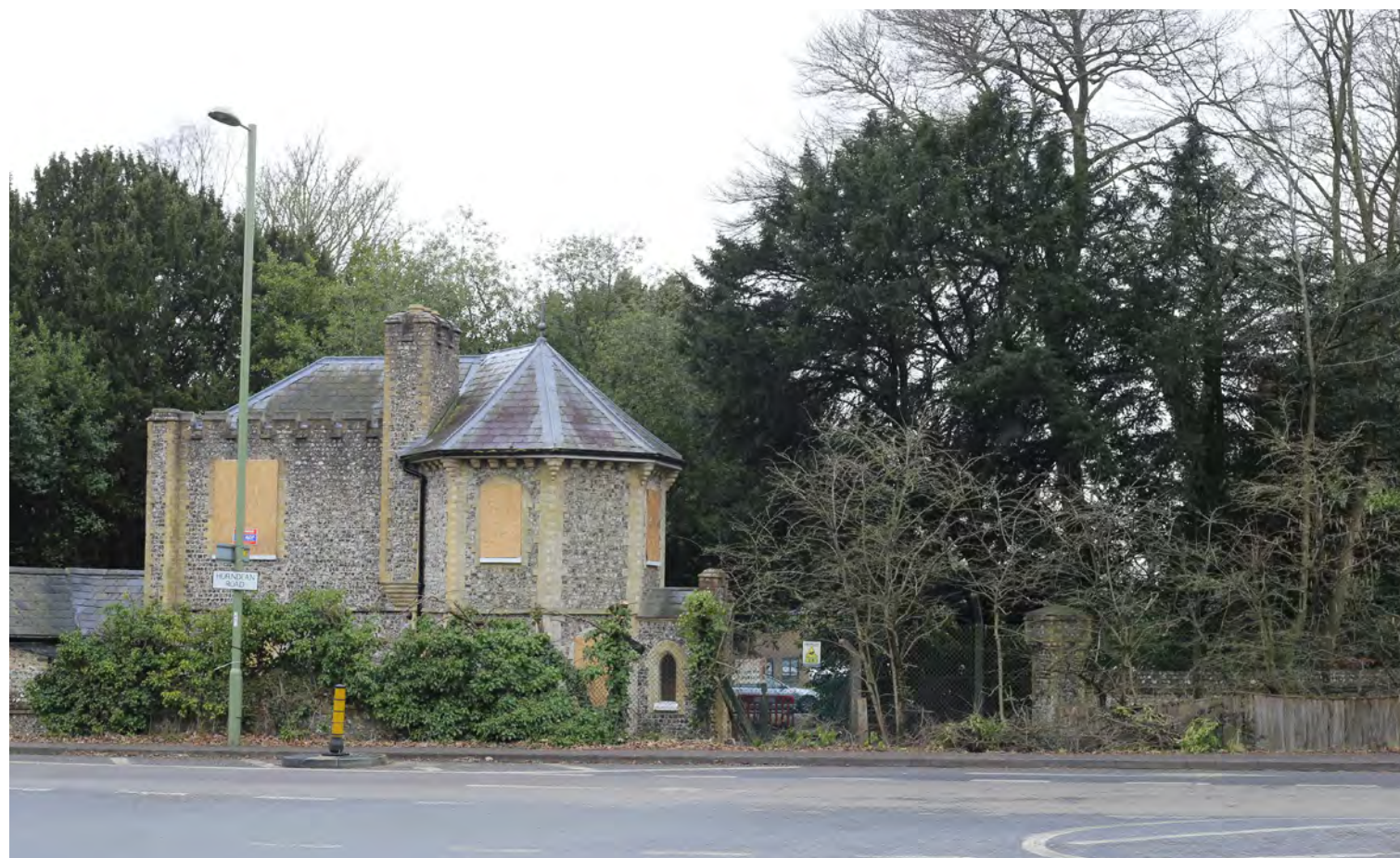
The entrance lodge on Horndean Road with the original access and part of the former northern boundary wall
