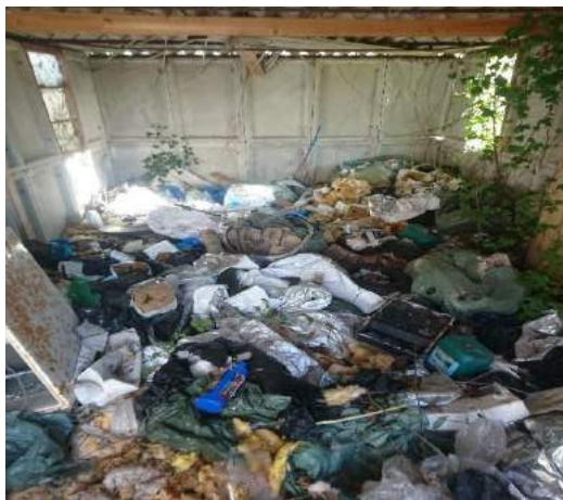
Existing internal garage state.
