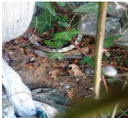
Concrete base showing after excavation.
