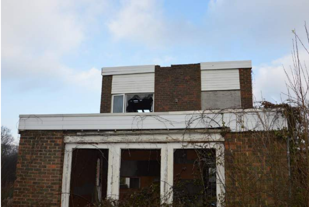
Plate 3. View of the south of the building.
