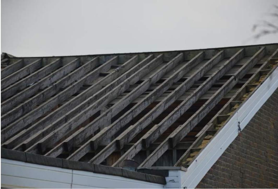
Plate 9. View of the exposed roof timbers and top of the wall.
