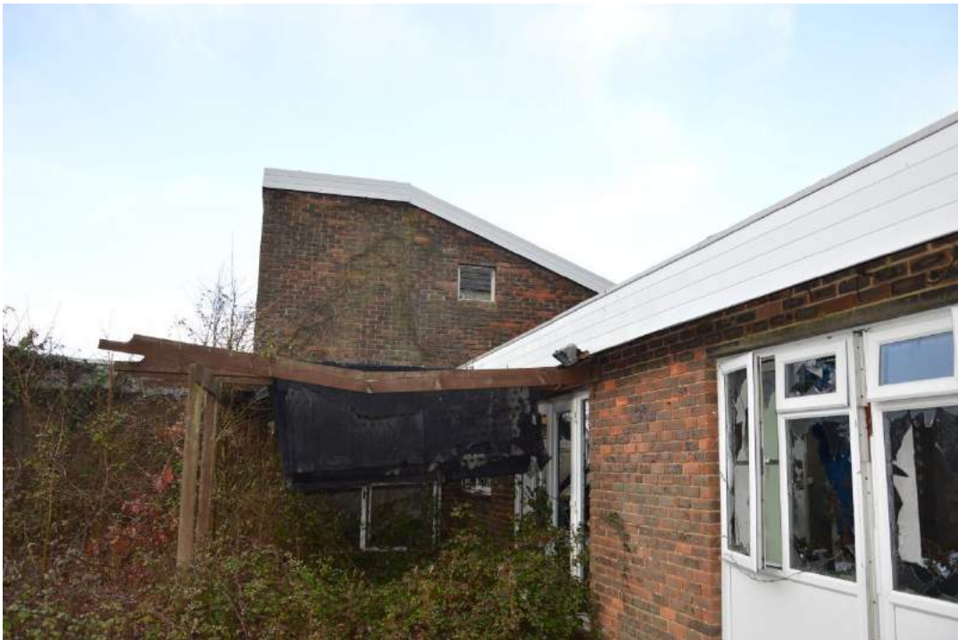
Plate 2. View of the south east of the building.
