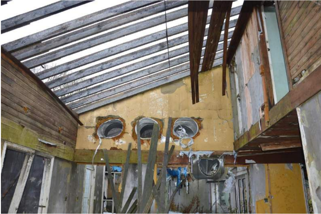
Plate 5. View of the interior of the building.
