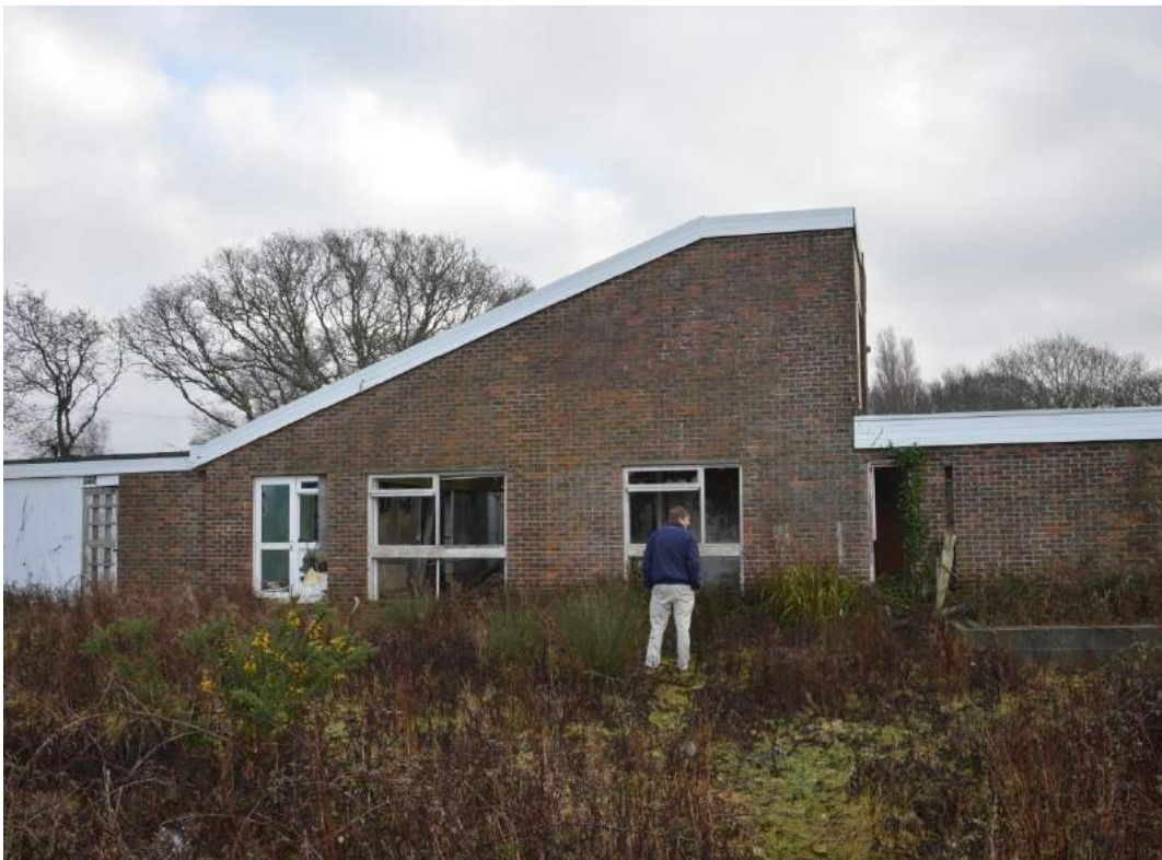
Plate 4. View of the west of the building.
