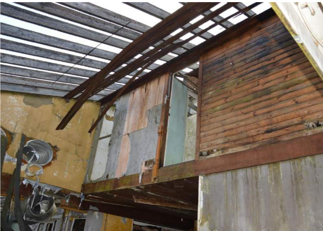
Plate 8. View of the interior of the building.
