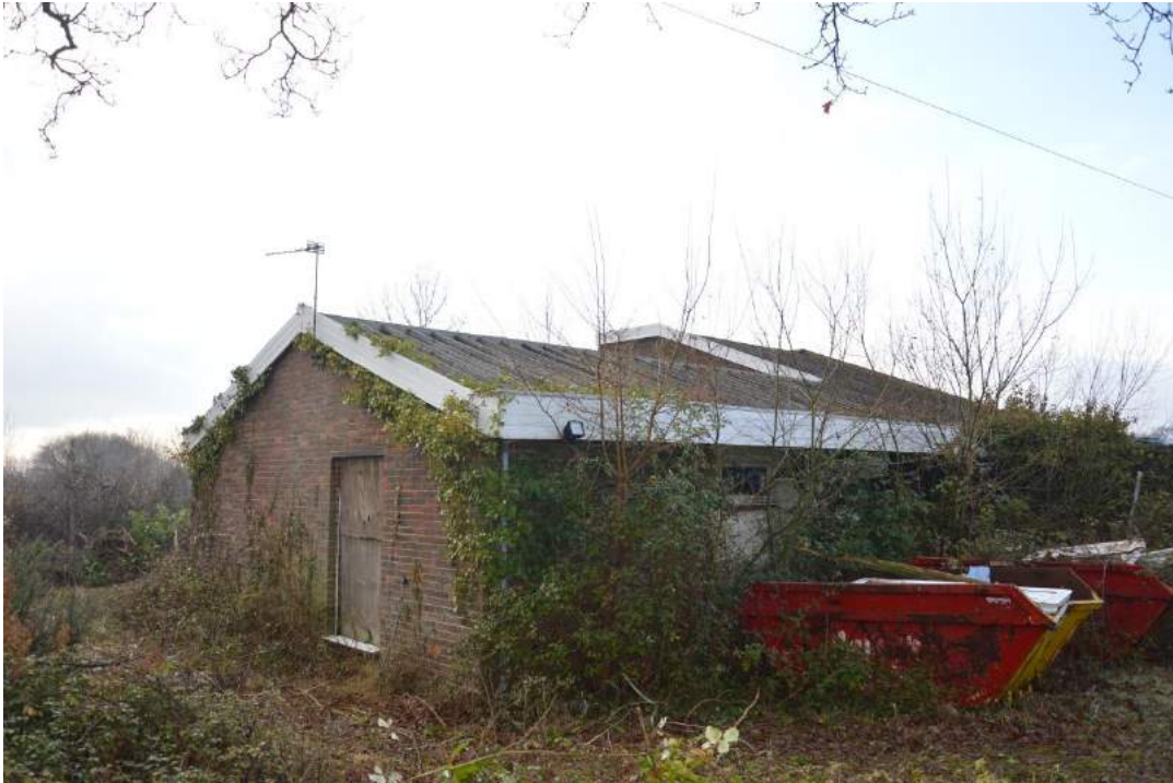
Plate 1. View of the north east corner of the building.
