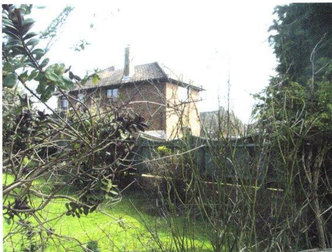
23 Warblington Road side elevation facing 2 Valetta Road
