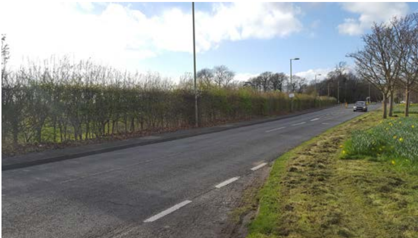
View north along Horndean Road with the site on the left
