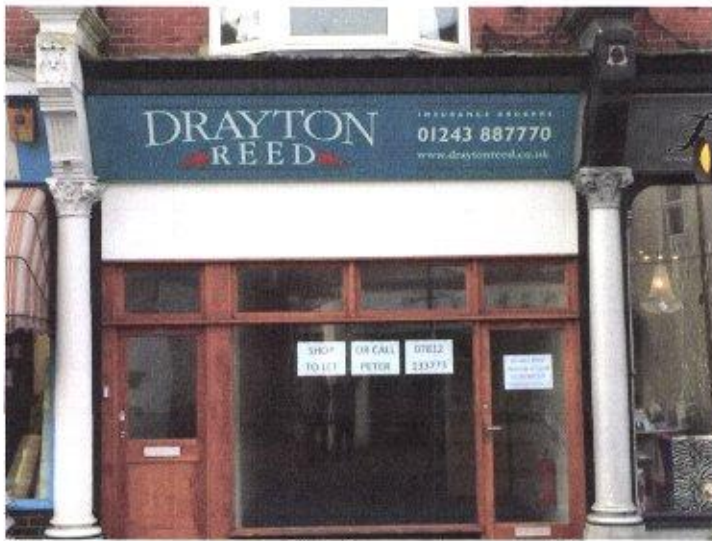
existing shop front
