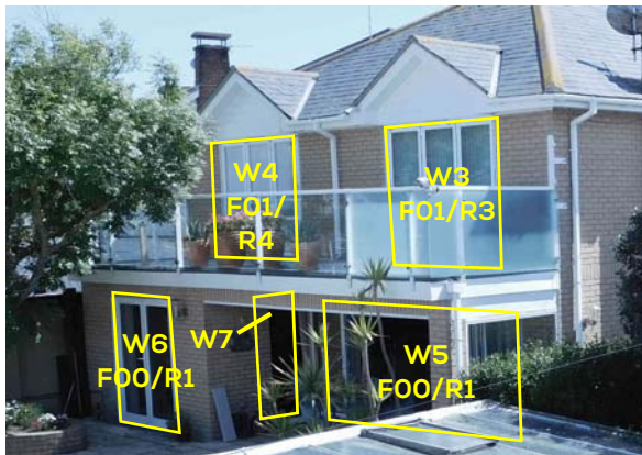
(Left) Rear of The Deck House
