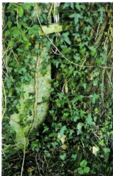
Figure 1. Eastern aspect of the stem compressed against the wall.
