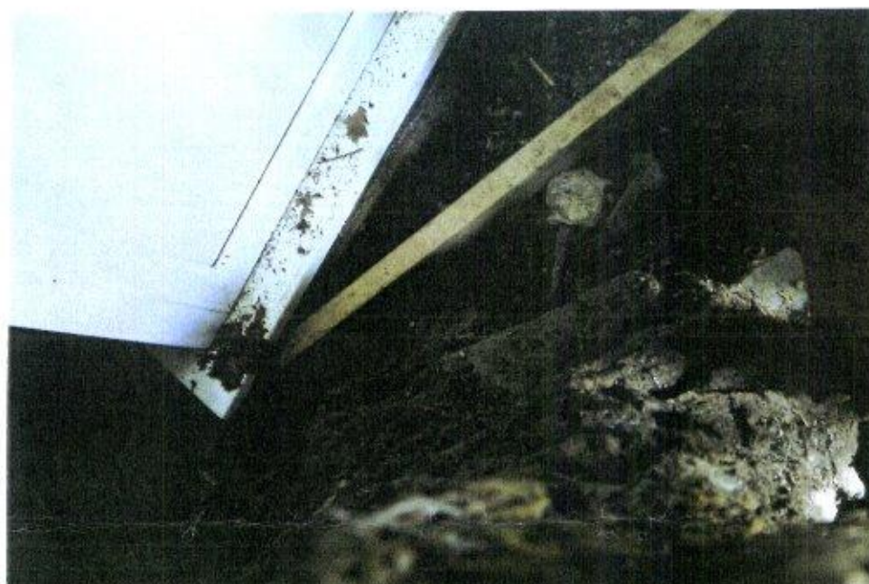
Figure 5. Looking down at the section of stem in the third property which could only be sounded with a mallet.
