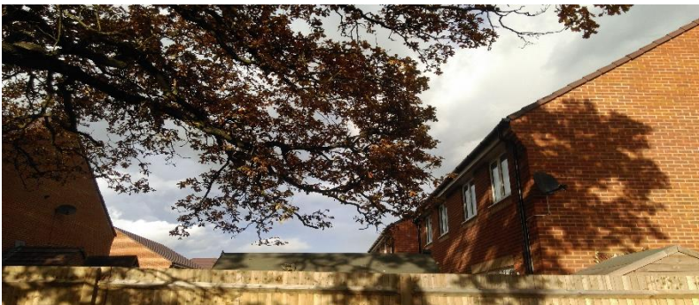
T56 Northern Crown Spread / Proximity to Building
