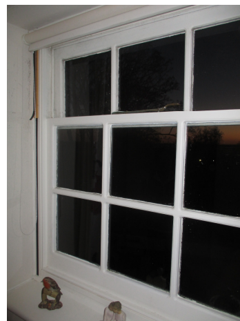
Fig 5 – Photo of existing second floor window with top sash being a top hung casement
