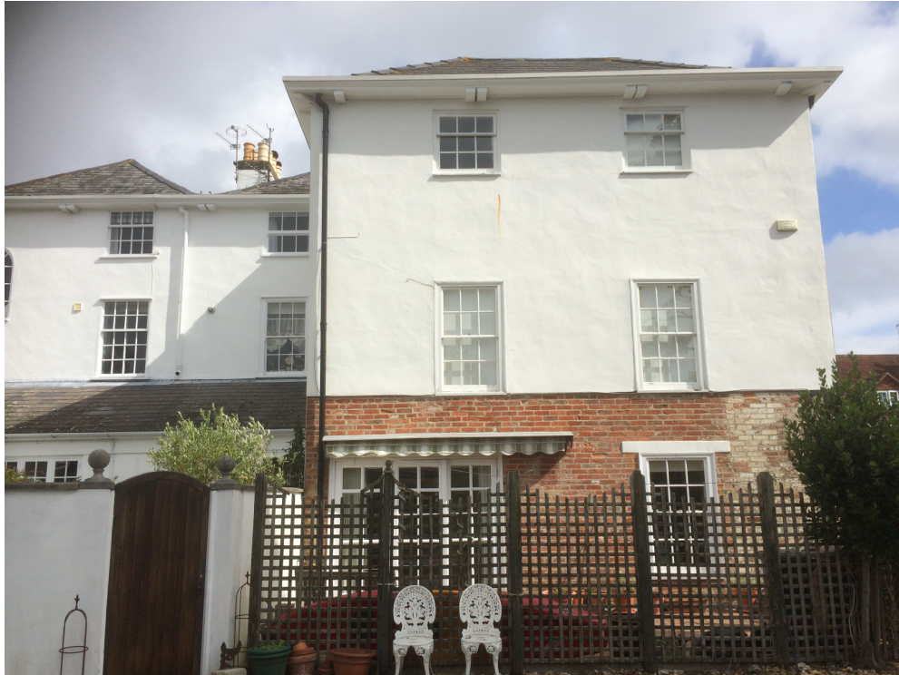
Fig 3 – Photo of the rear of the property also showing the rear view of 5 Kings Street (behind to the left), with original sash windows with horns and no external architrave around the frame.
