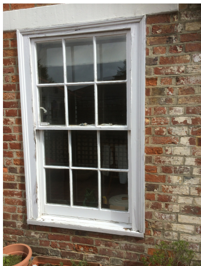
Fig 3 – Photo of typical timber sash window
