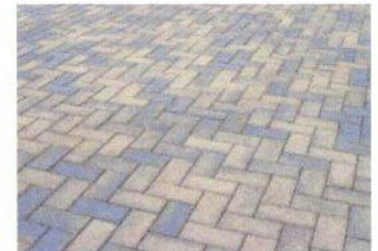
Brickette hardstanding for car parking
