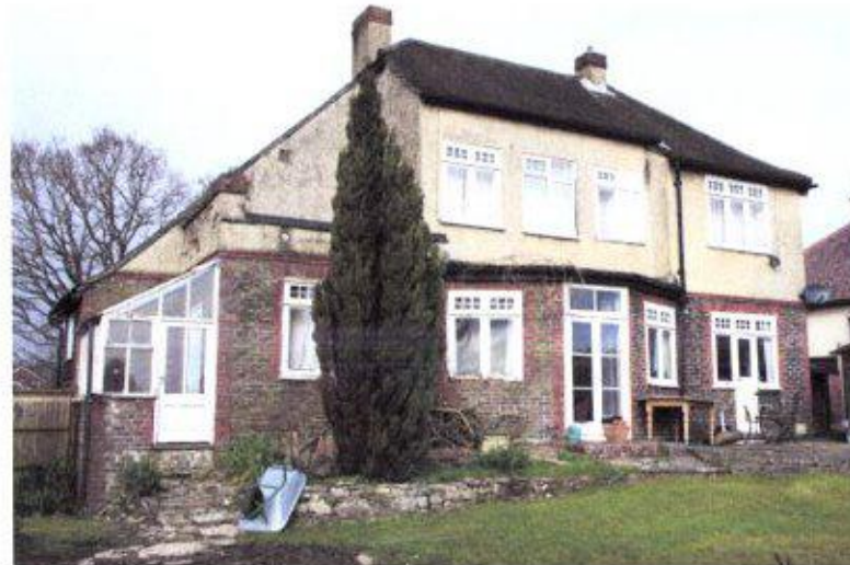
5. Rear elevation of existing house
