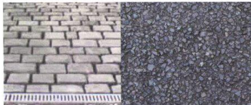
Cobble rumble strip at entrance and permeable tarmac access drive
