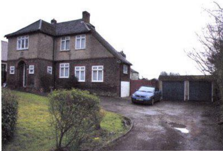
1. Front elevation existing house
