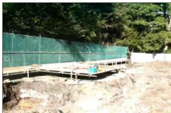
Ground protection image 4: A scaffold framework attached to the main scaffold fencing can be used to support either scaffold planks or plywood to create an elevated platform with a gap beneath.
