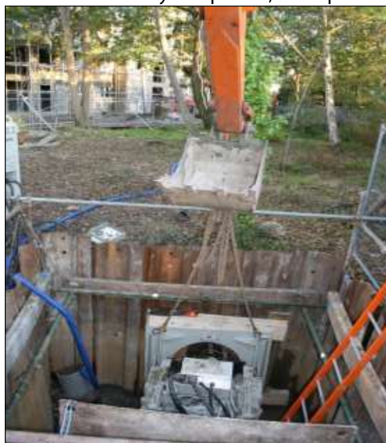
Services image 1: If possible, thrust boring is the preferred option for installing service routes through the RPAs of important trees, but there has to be space at the start and finish to dig substantial working pits.
