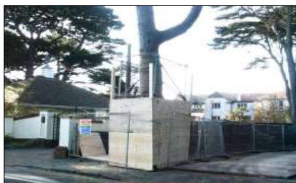
Fencing image 6: Board secured to scaffold framework adds another layer of protection for vulnerable trunks and branches
