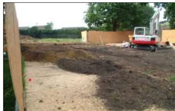
Ground protection image 2: Spreading soil excavated from footings is an effective way of buffering the plywood surface from the wear of light vehicles.
