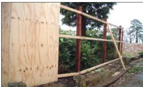
Fencing image 4: Board specification on secure wooden posts is a suitable alternative to the standard braced scaffold design.
