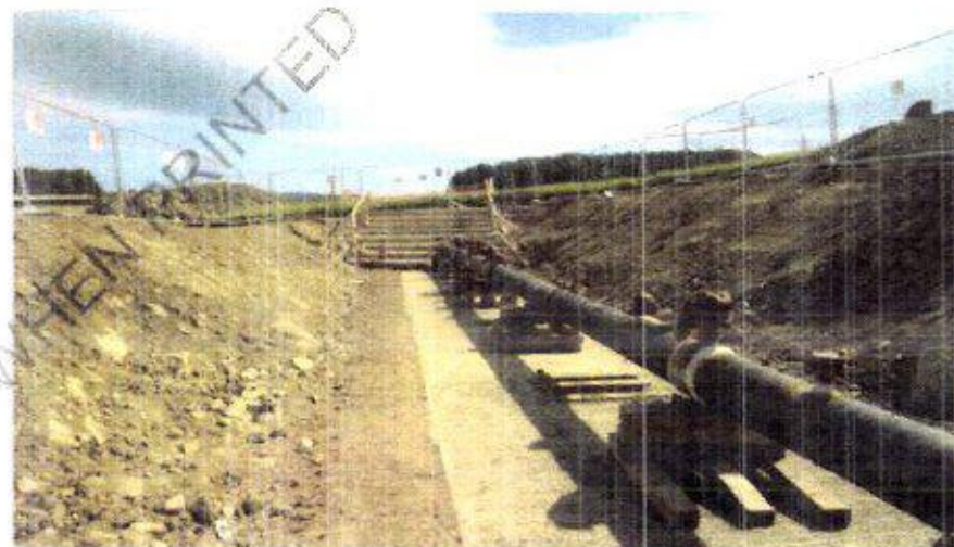
Figure 20. Pipeline Supports
