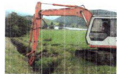
Figure 2. Ditch Maintenance
