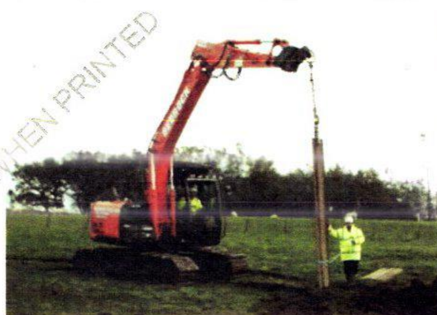
Figure 21. Example Lifting Operation
