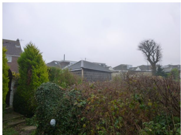
The subject building viewed from the northwest, on Wayfarers Walk.
