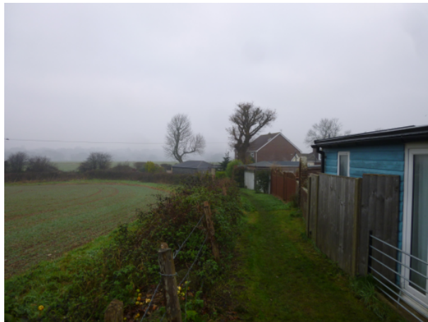
The subject building viewed from the south on Wayfarers Walk.
