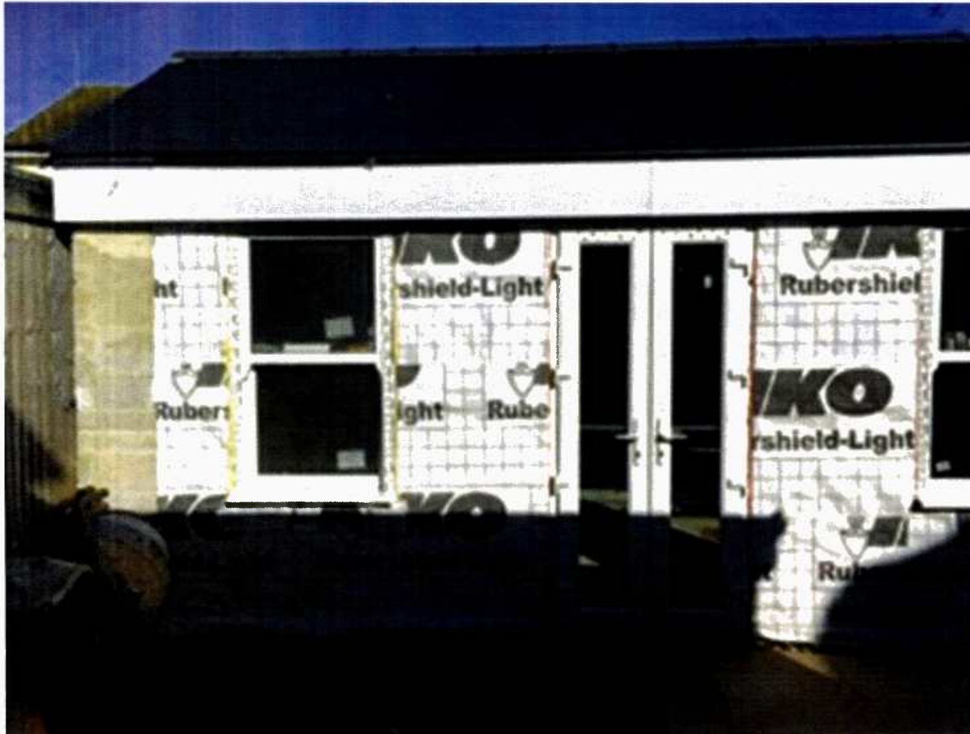
West elevation – as built 1
