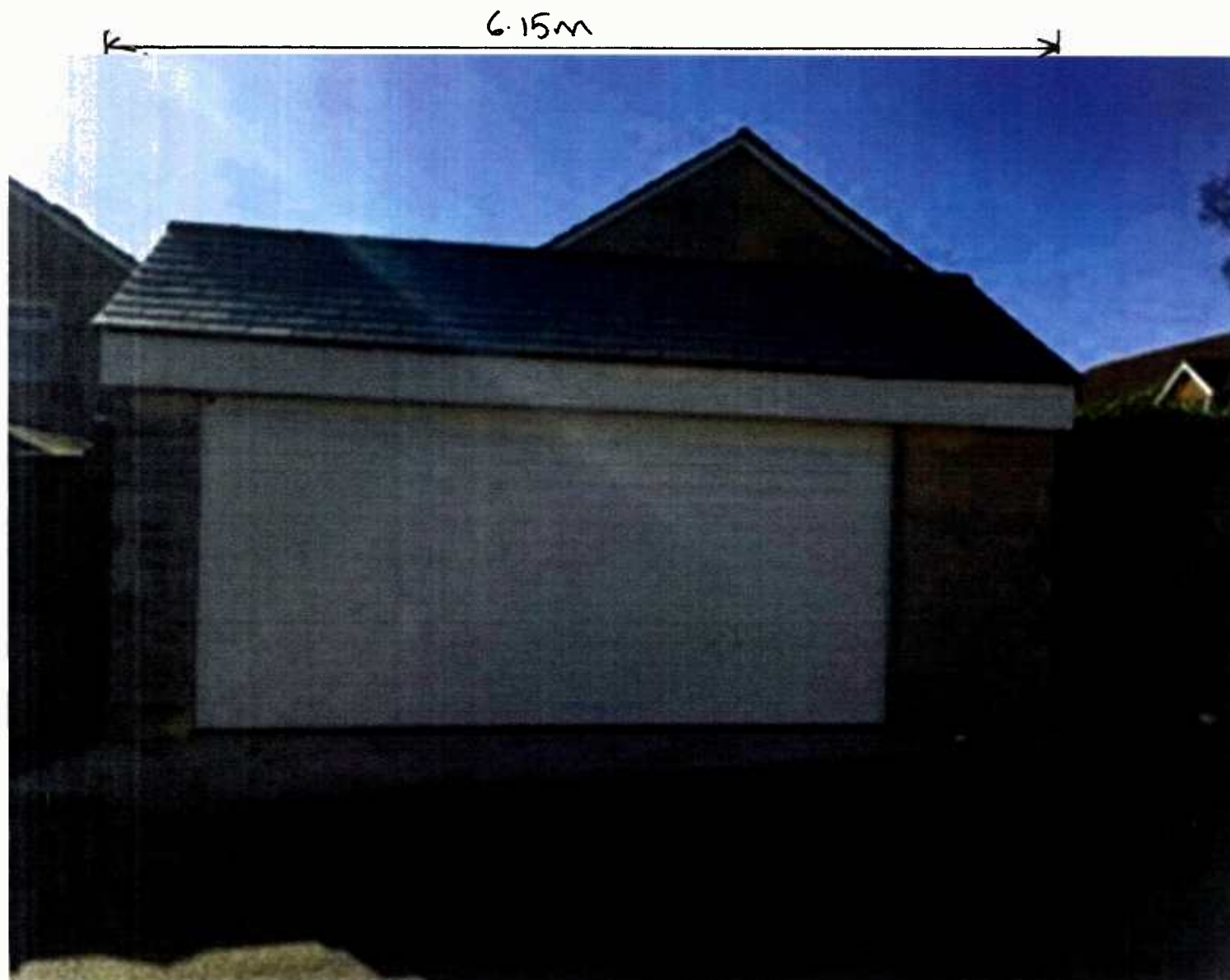
East elevation – as built
